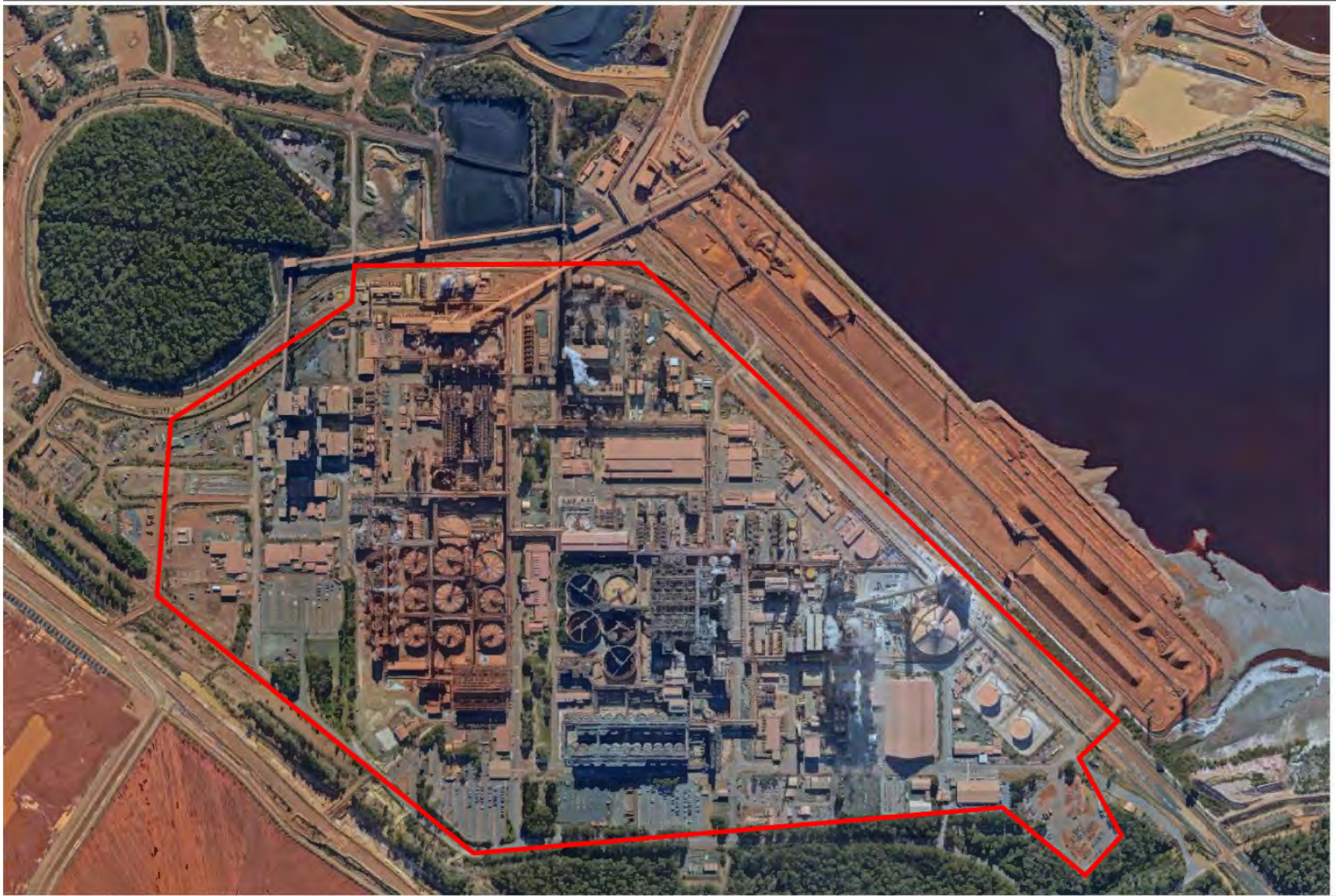
Figure 3-3: Recent satellite image of the processing area on the prescribed premises
