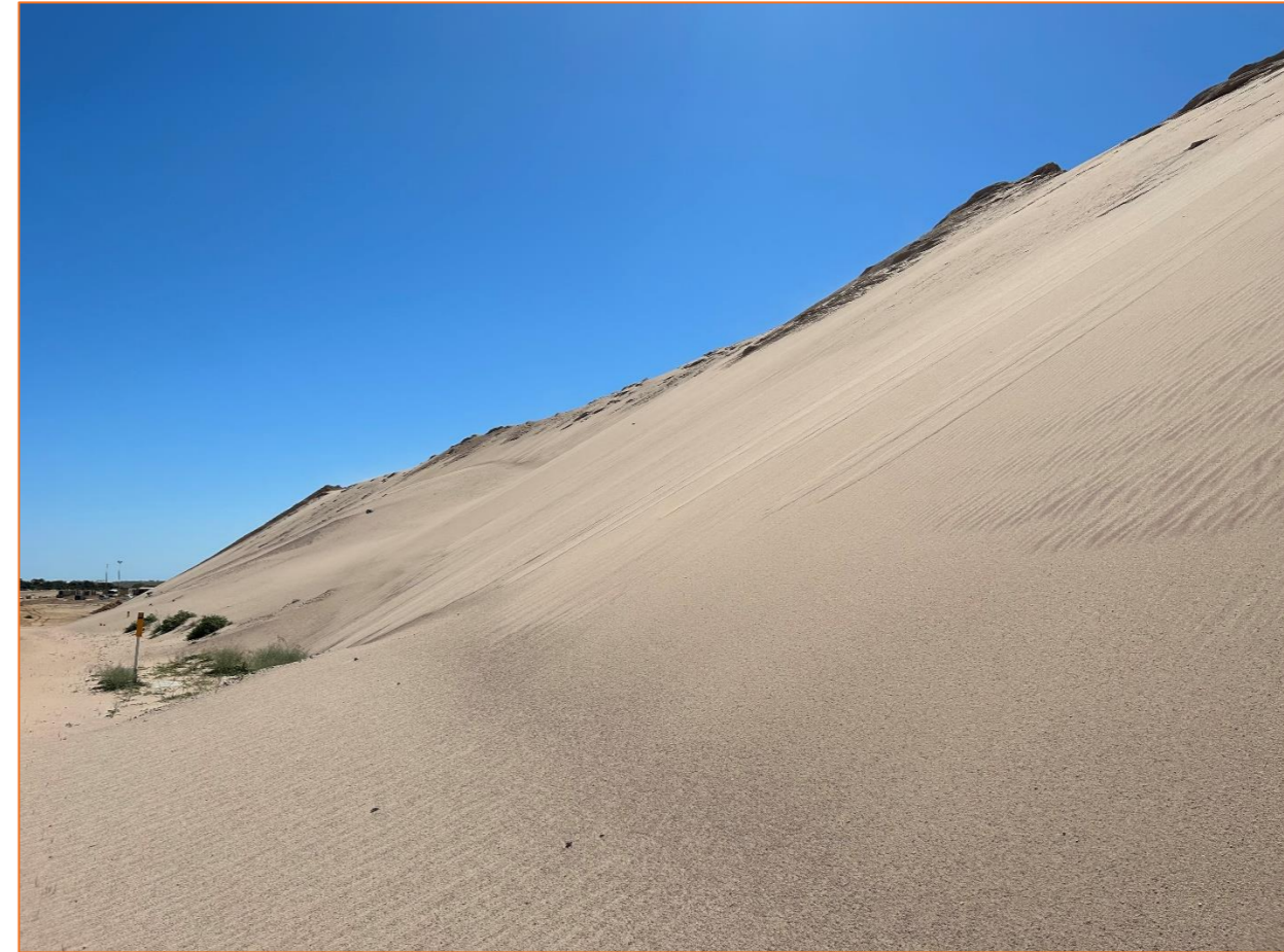
Figure 3-3: Dry tailings storage facility – close view of western face (ETA, 2023)
