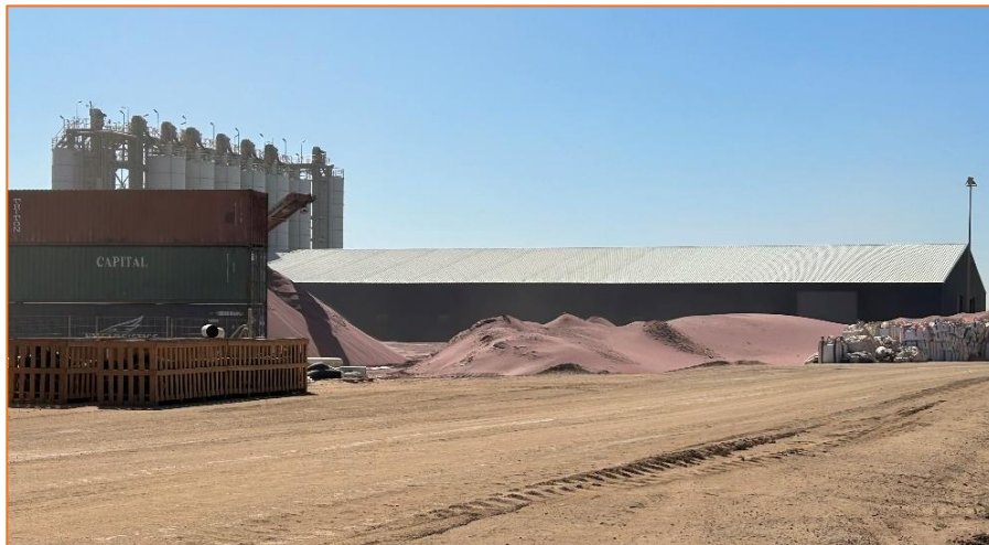
Figure 3-10: Product stacking protected by stacked shipping containers (ETA, 2023)
