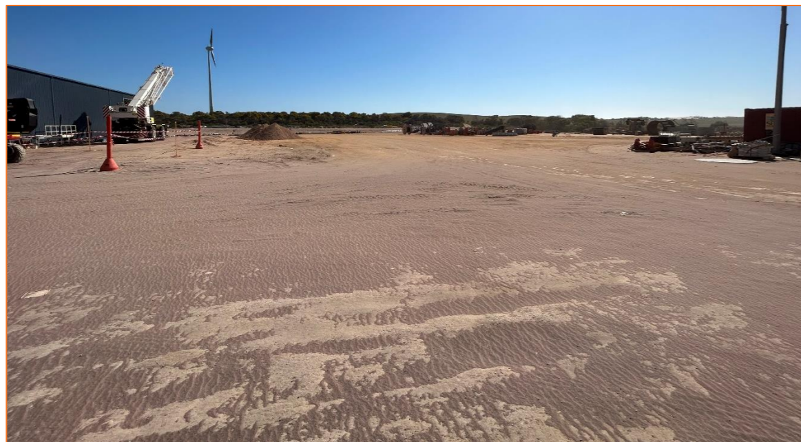
Figure 3-8: Open areas near ilmenite shed and laydown yard (ETA, 2023)
