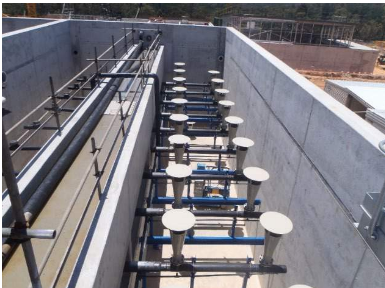
Plate 17 - Example of an ActiDAFF® Cell during Construction (Northern Water Partnership, 2023)
