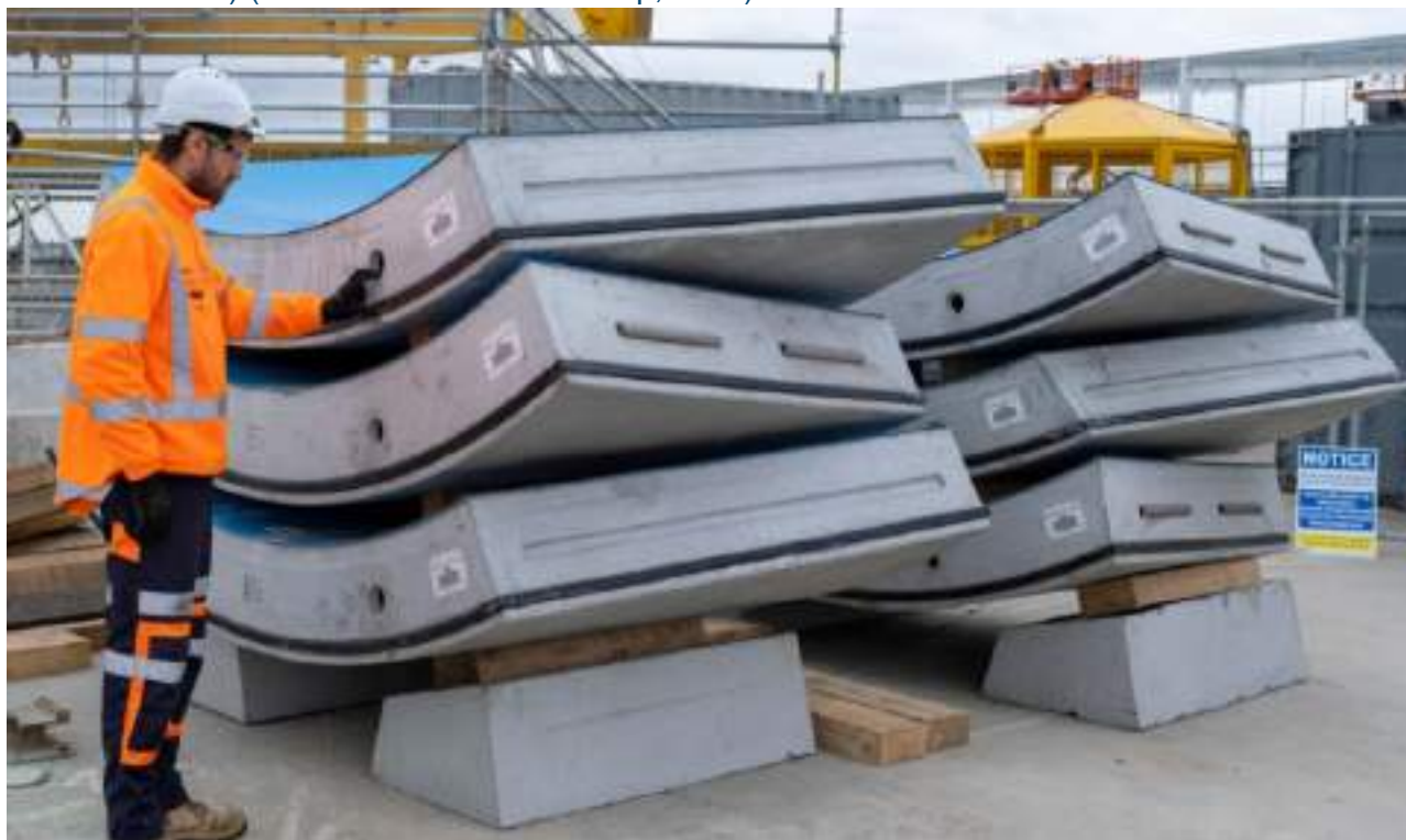
Plate 8 - Example of Typical Pre-cast concrete tunnel segments with single seal (Northern Water Partnership, 2023)
