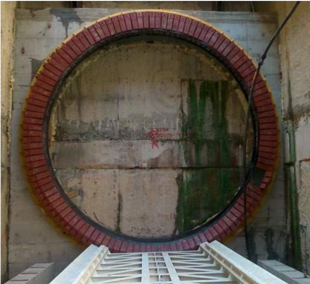
Plate 7 - Typical TBM Launching Pad and Sealing Ring (Northern Water Partnership, 2023)
