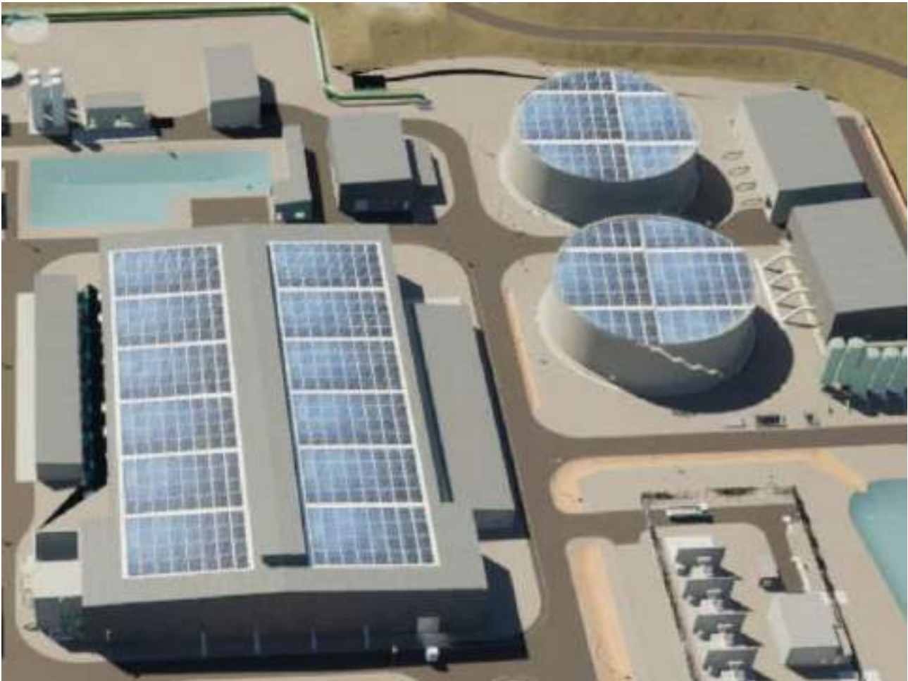
Plate 35 - 3D Model of Rooftop Solar on Stage 1 RO Building and Drinking Water Tanks (Northern Water Partnership, 2023)
