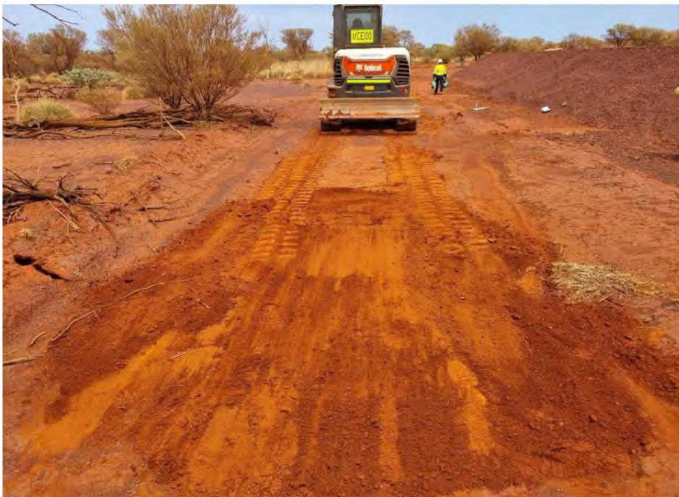
RR-TPG02 After Reinstatement
