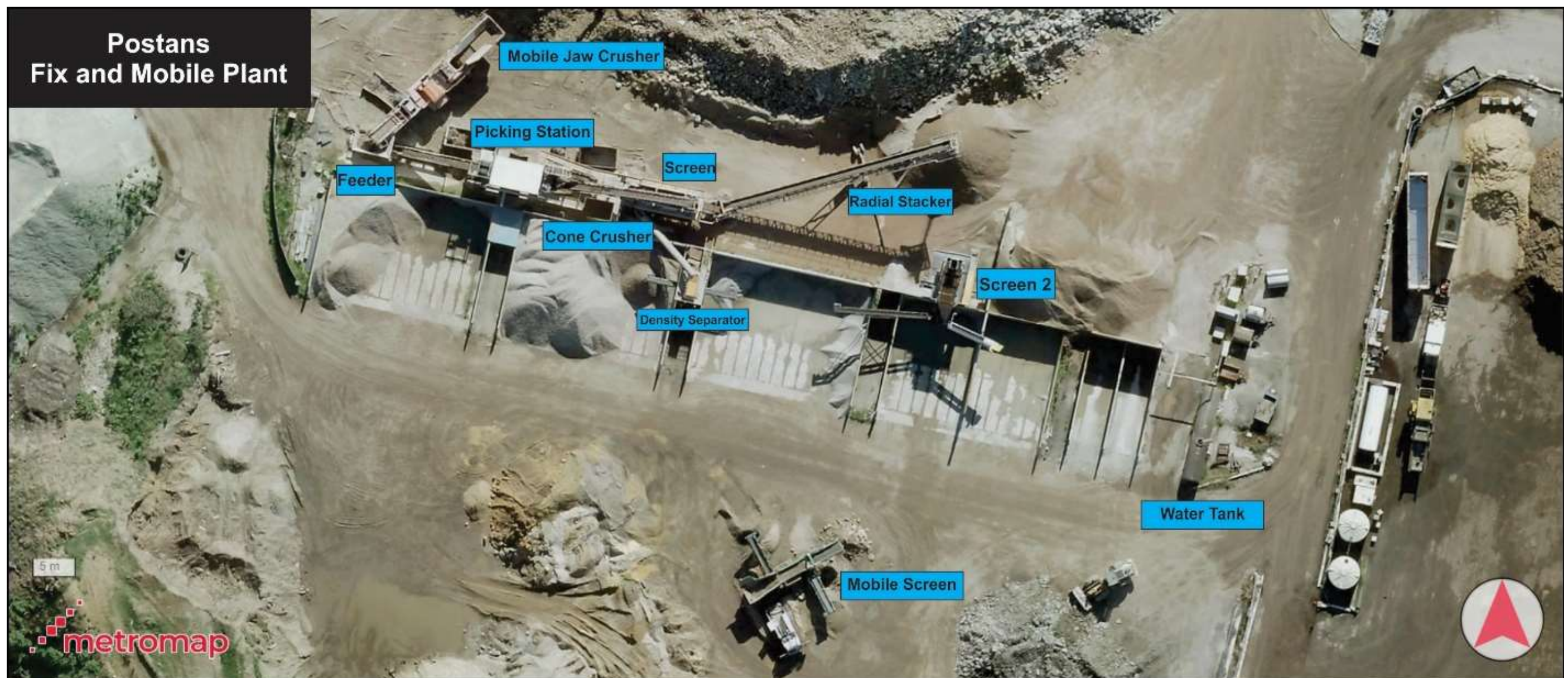
Figure 3: Location of fixed and mobile picking, crushing and screening plant
