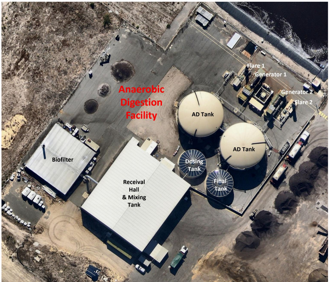
Figure 3: Anaerobic Digestion Facility
