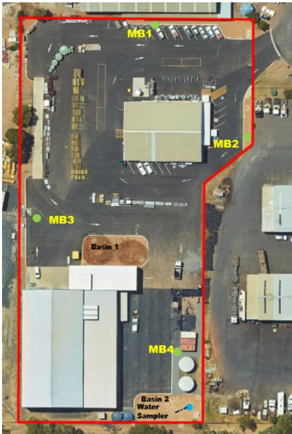
Figure 3: Ambient groundwater monitoring
