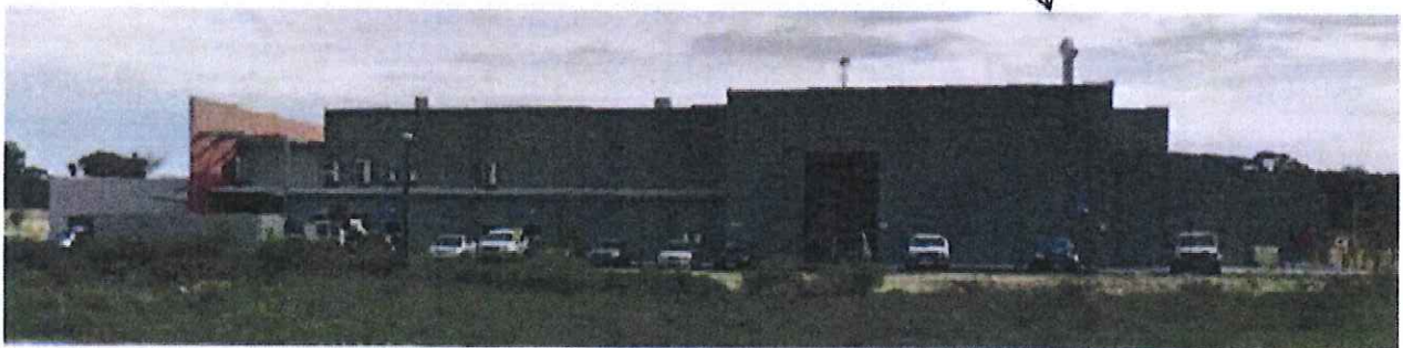
Elevation taken from Greenwich Parade showing Eastern side of building.
