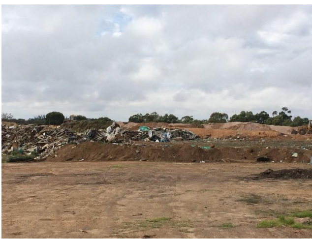
Photo 3 – Uncovered waste in landfill area
