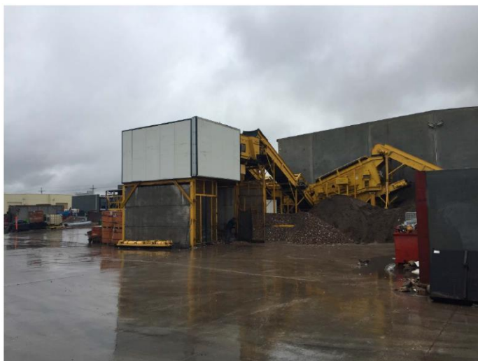
Figure 6: End of machinery barrier
