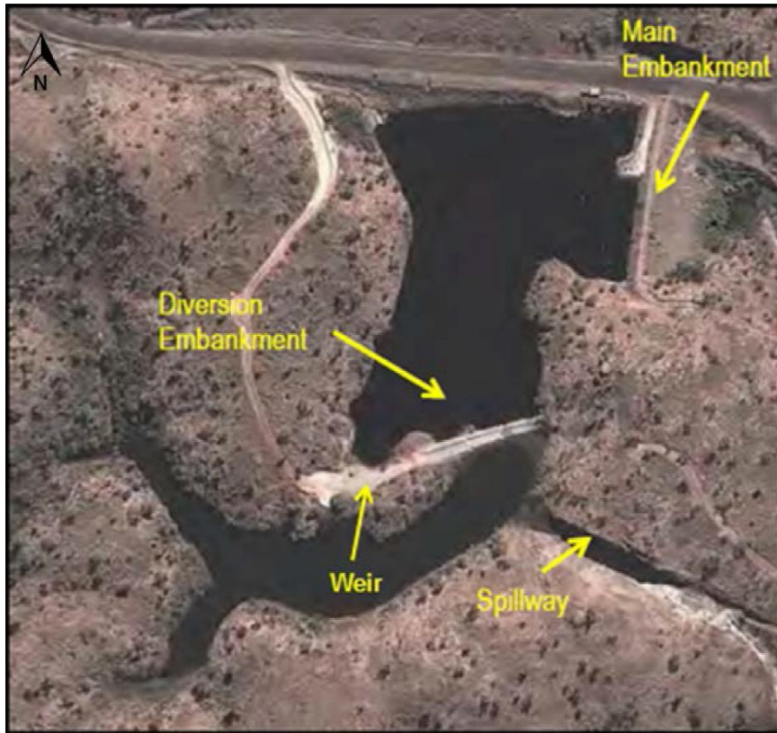
Figure 1: WSF1 and Spillway
