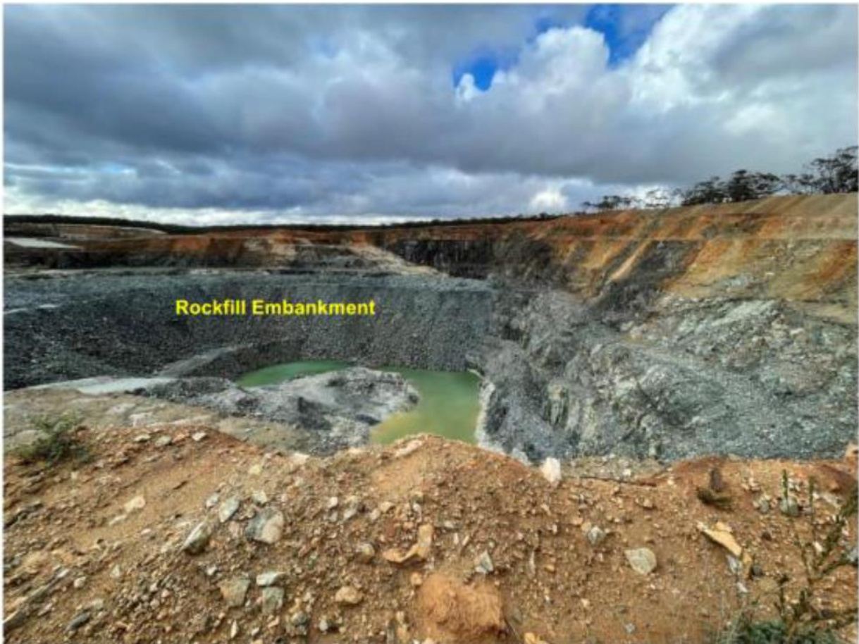
Figure 1: Location of the rockfill embankment which sections off a portion of the 2SE pit for tailings storage.
