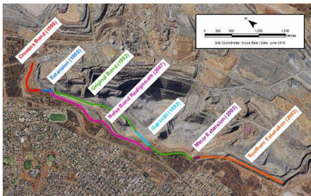
Figure 2: KCGM Environmental Noise Bund Construction History
