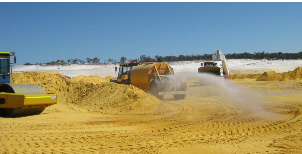
Plate 4: Water truck for dust suppression
