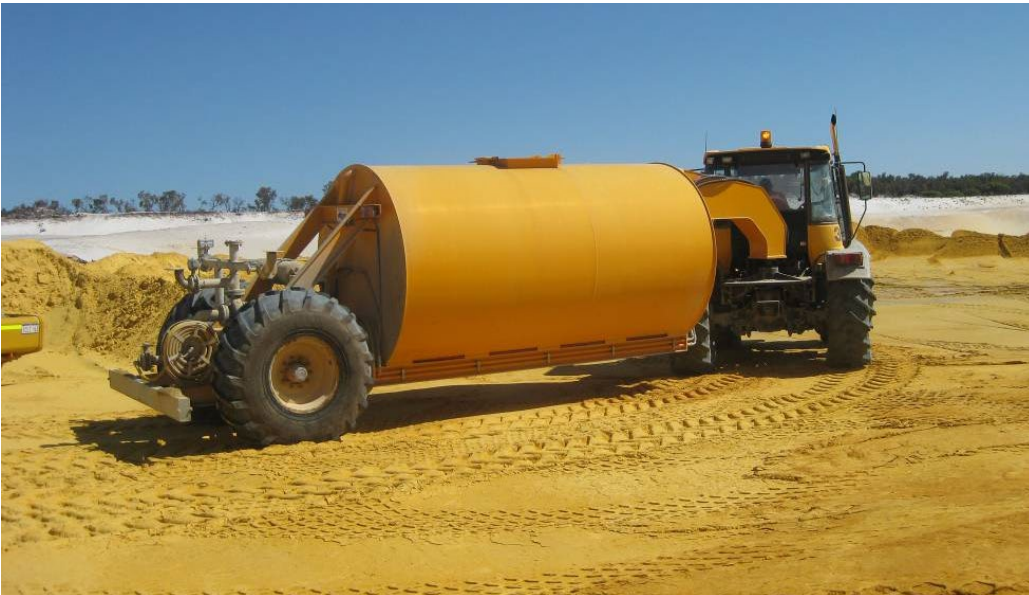
Plate 3: Water truck for dust suppression
