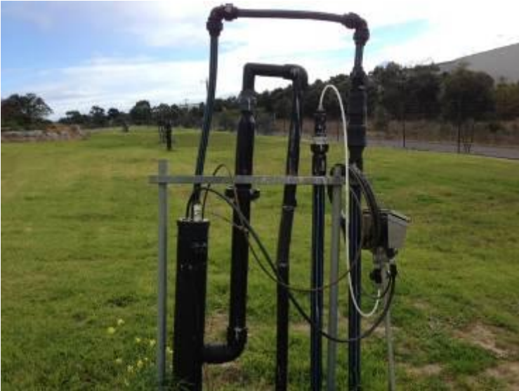
Combined Leachate and Gas Extraction Well Head
