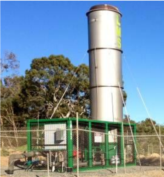
Large 2,000m 3 /hr fully enclosed flaring unit
