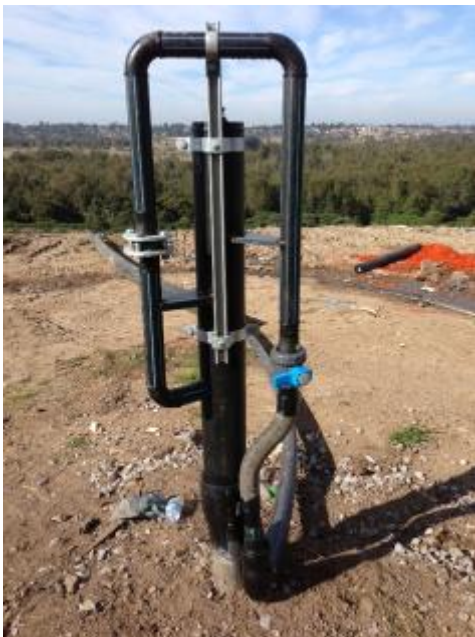
Basic Well Head Arrangement
