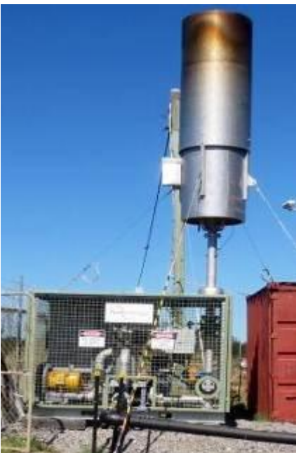
Large 2,000m 3 /hr fully enclosed flaring unit
