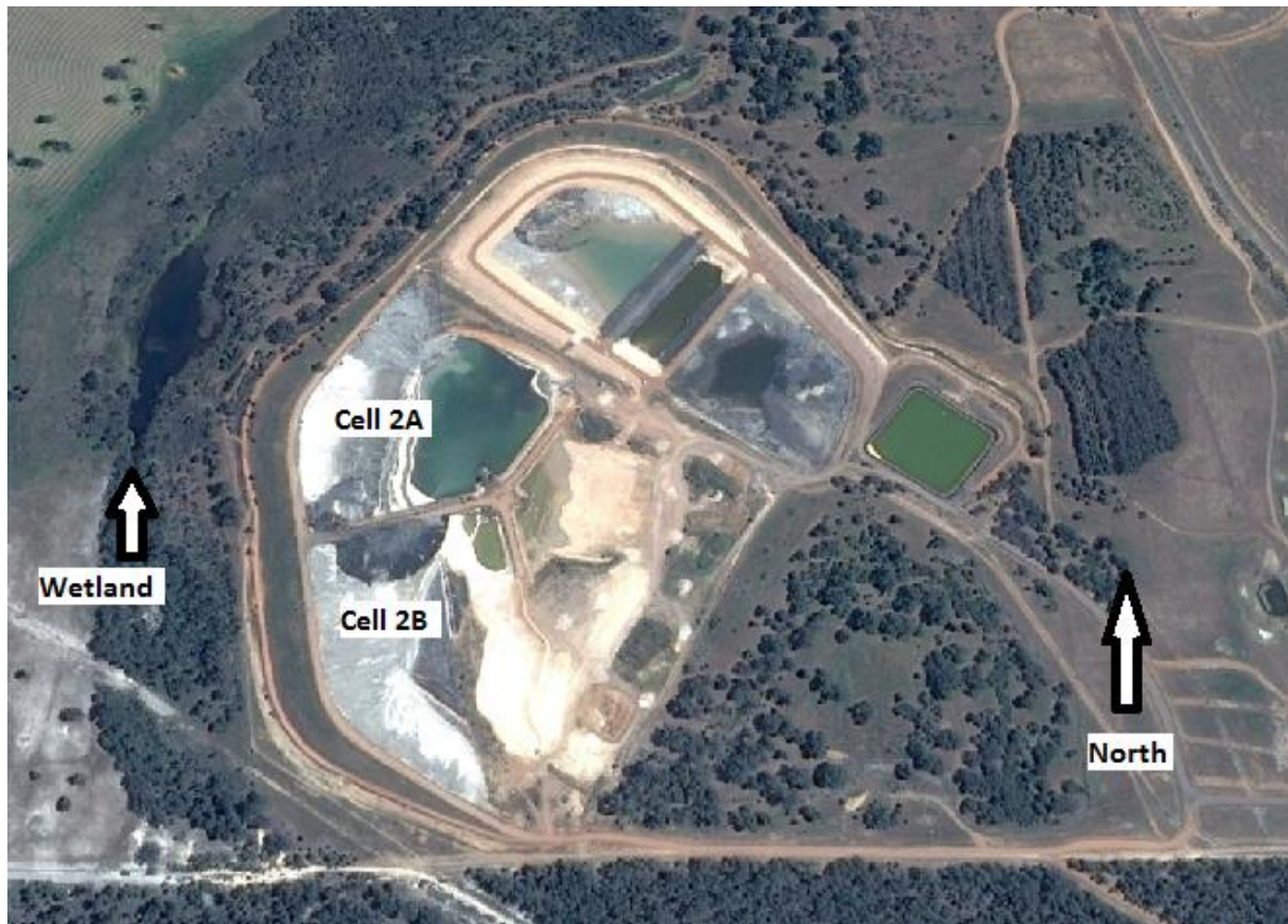
Figure 3 Location of wetland area downstream of flyash dam
