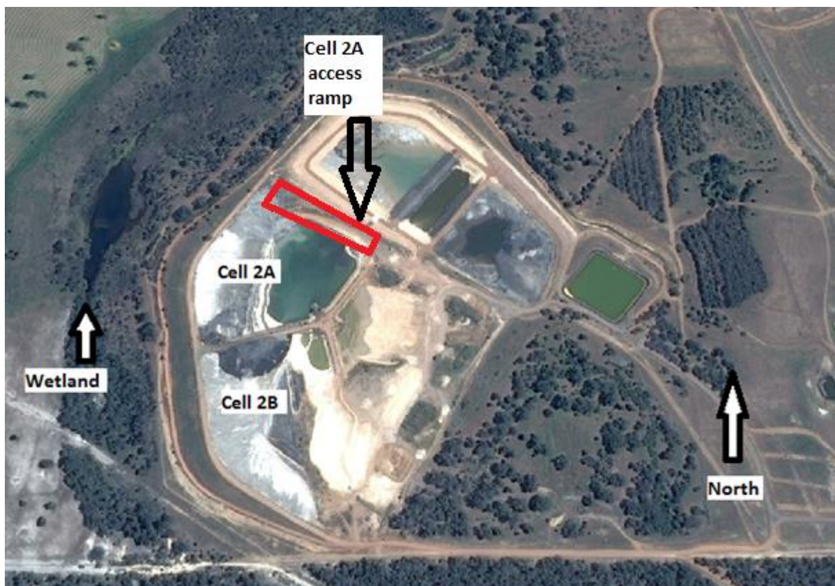
Figure 1: The Collie 'A' Power Station Flyash dam access ramp
