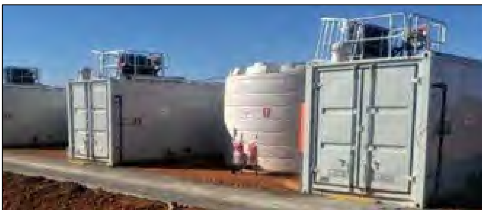
Figure 2:1 Example SBR WWTP (4 x process trains)
