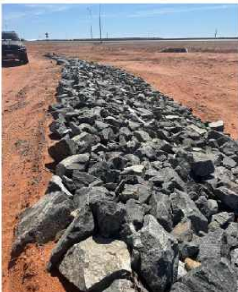
Pond 5 Emergency overflow with rock armour embankment protection. Surface flow to NW Hwy culvert in rear of image
