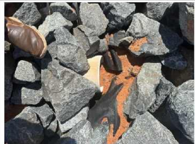
Pond 5 Emergency overflow pipe on external embankment with rock armour embankment protection.
