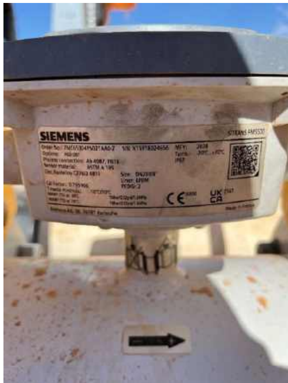
Figure 1.5 Turkey Nest Discharge Flowmeter Details
