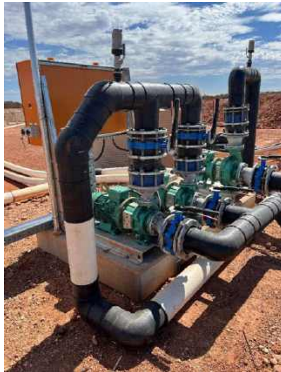
Figure 1.2 Mesa Transfer Pumps
