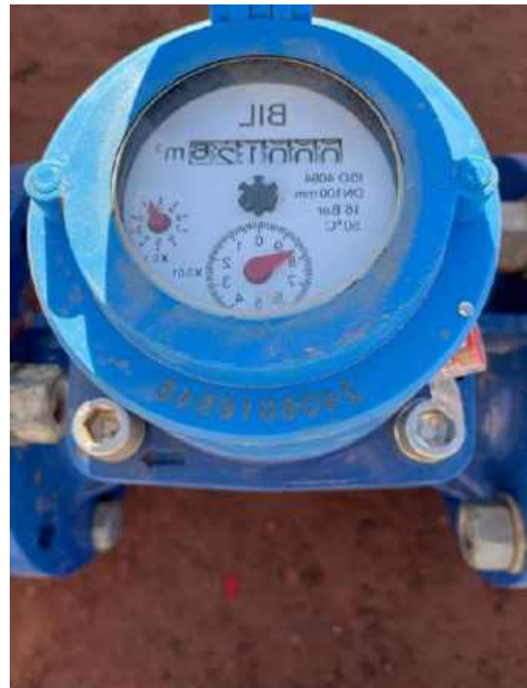
Figure 1.6 Central Pit Abstraction Flow Meter Details
