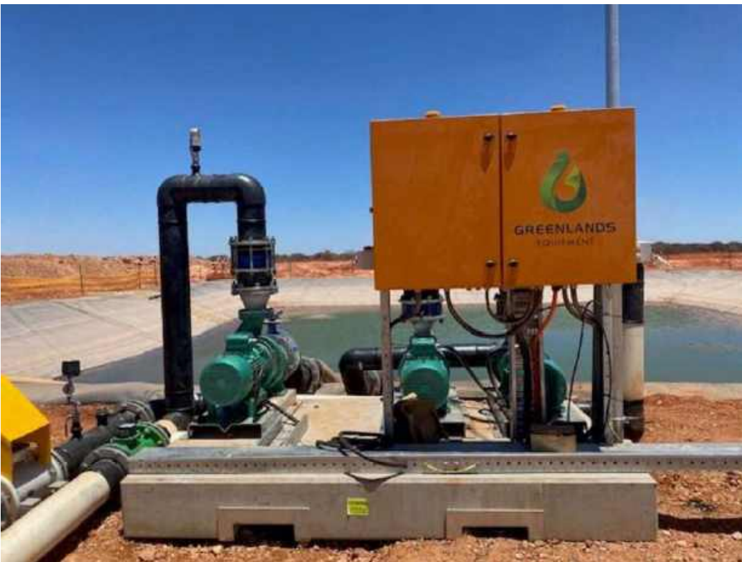
Figure 4: Telemetry Box, Pump and Metering Set-Up for Standpipe Line (right) and Mesa Discharge Lines (left)
