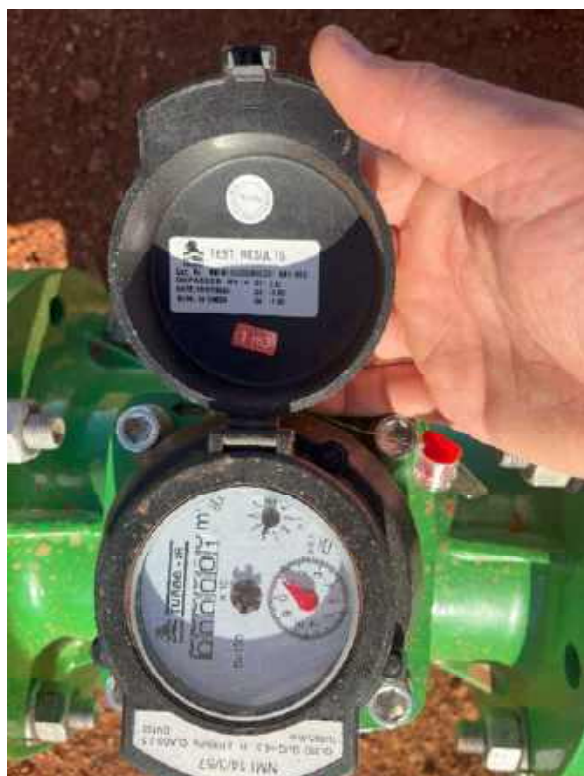
Figure 1.7 South Pit Abstraction Flowmeter Details
