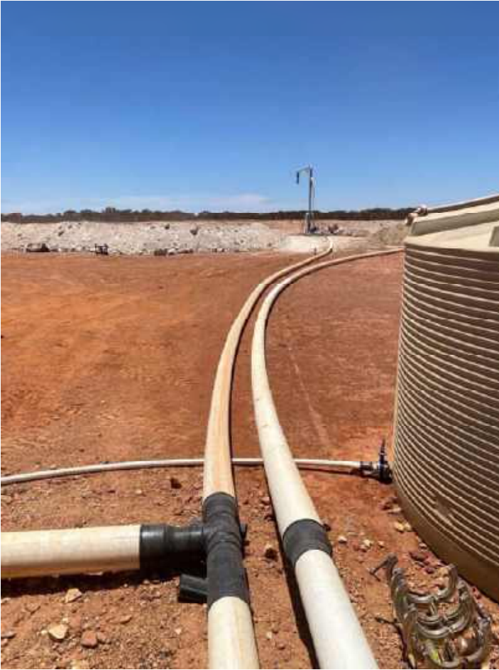
Figure 3: Dewatering from Turkey Nest - Standpipes Line (left) Mesa Discharge Line (right)
