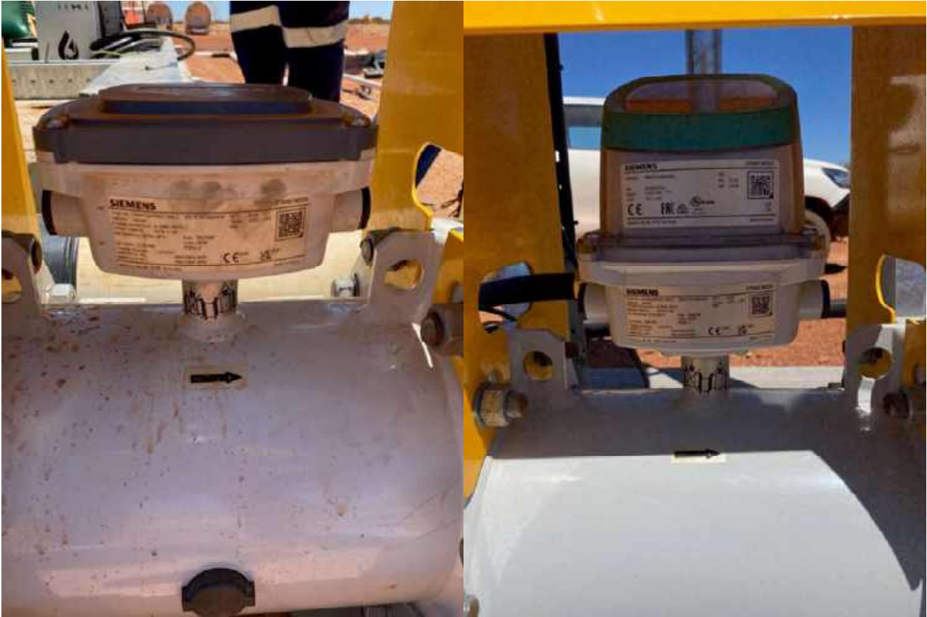
Figure 5: Magnetic flow meters for Telemetry - Turkeys Nest End (left), Mesa Discharge End (right)
