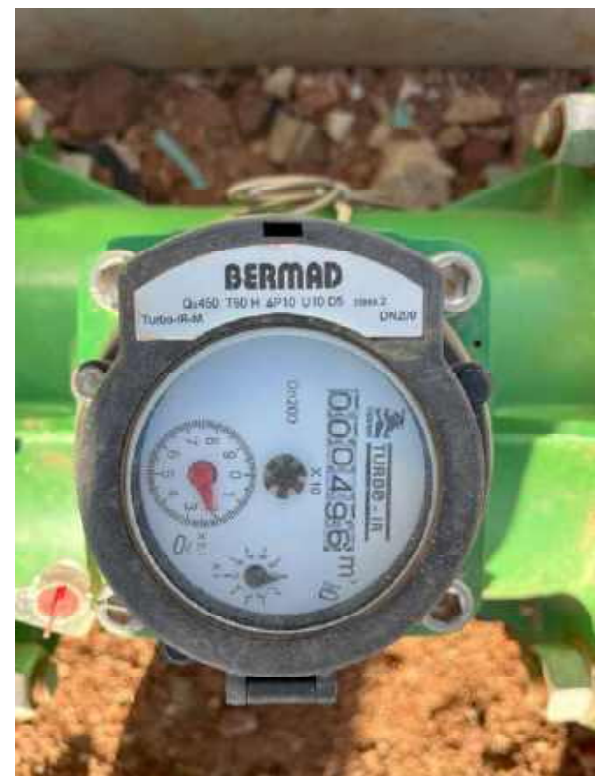
Figure 1.8 Standpipe Discharge Flowmeter Details-1
