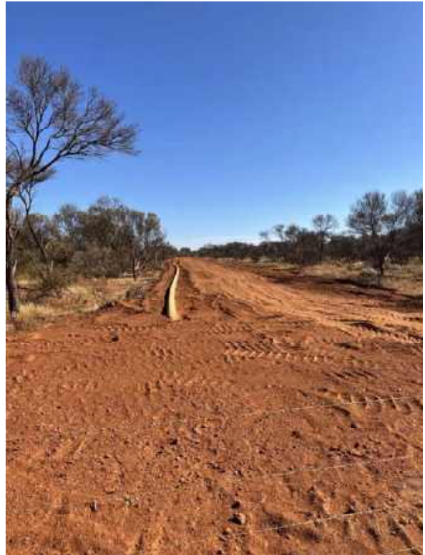
Figure 1.10 Mesa Transfer line in V-drain
