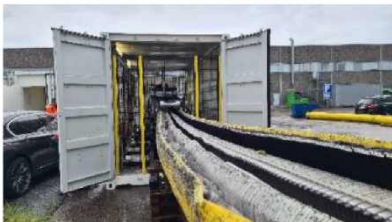
Flexible pipe being de-tension by cutting
