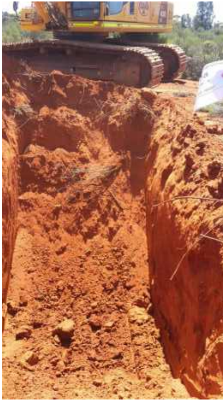
Plate 158: Test Pit TP-29
