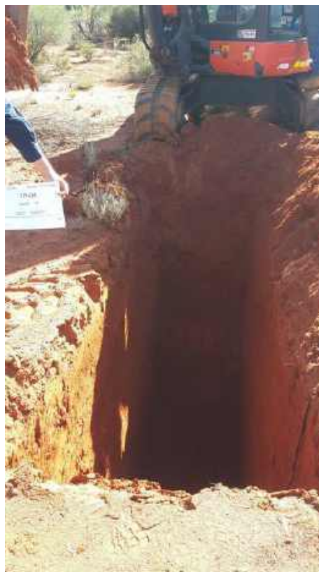
Plate 17: Test Pit TP-04
