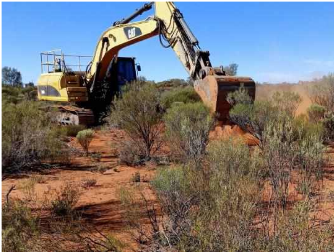
Plate 237: Test Pit TP-47
