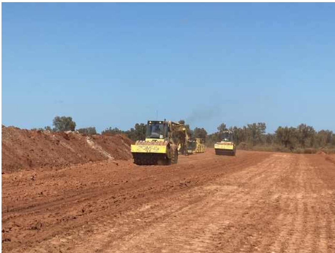
Plate 3: Compaction Zone C material, Cell 3 - North embankment, Layer – 2.
