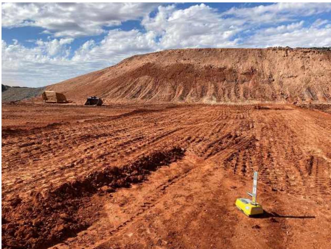
Plate 4: NDM Compaction test at South Embankment – Zone C – layer 1.
