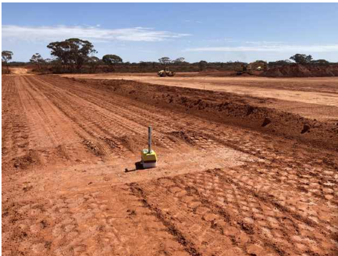
Plate 4: Field Density Testing, Cell 3 – West embankment, Layer – 3.
