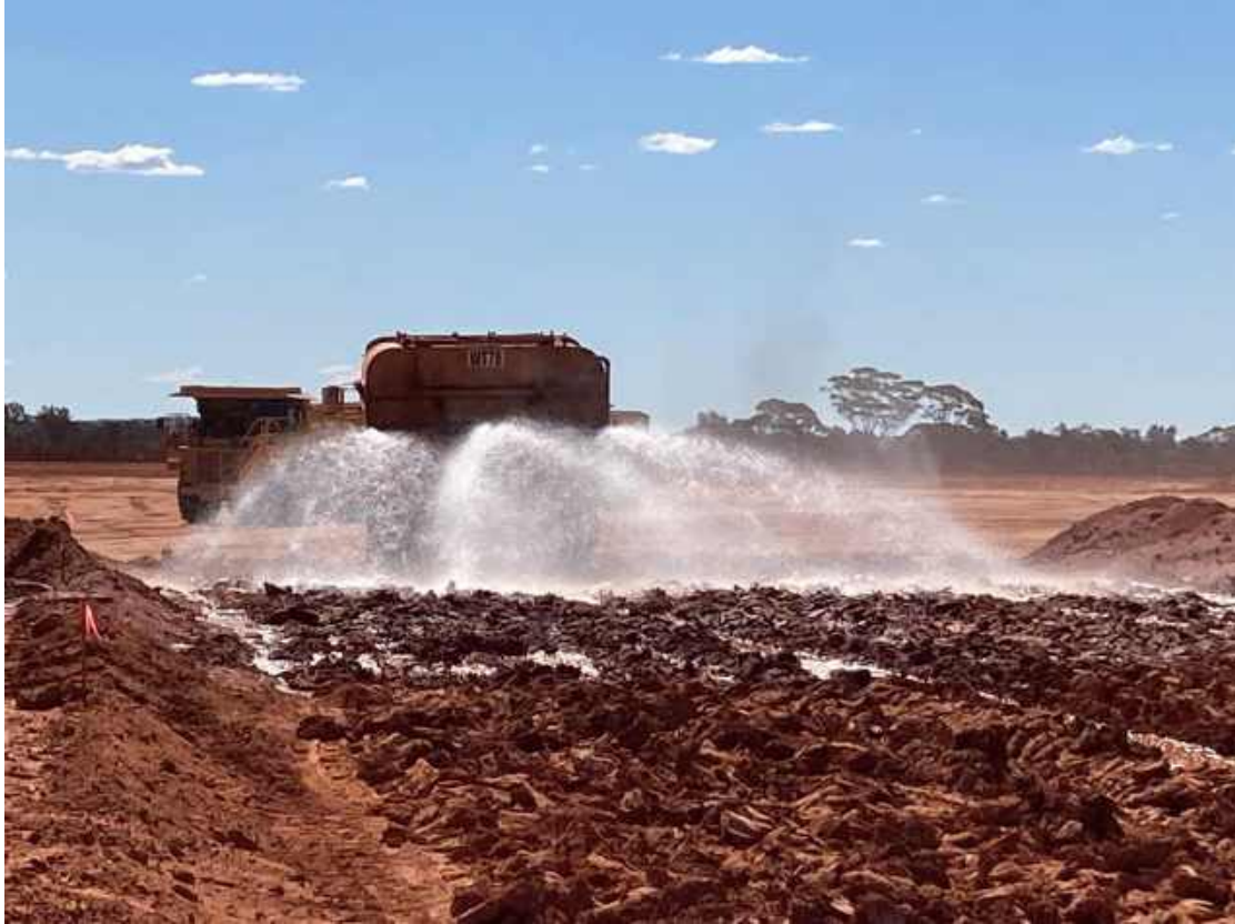
Plate 5: CSL Trial Pad moisture conditioning with water truck.
