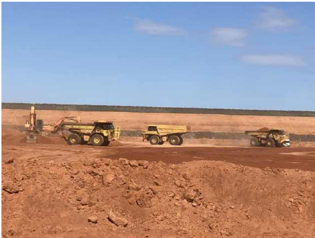
Plate 1: Loading Zone C material at borrow pit.
