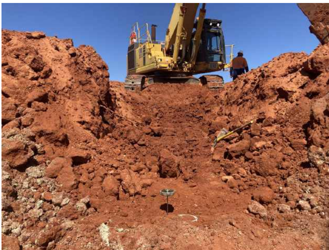
Plate 6: UD sampling at North embankment Cut-off trench (3.0m depth), for Laboratory Shear test
