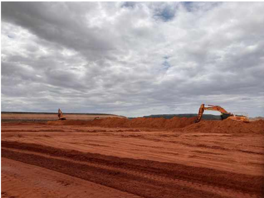
Plate 4: Excavating Decant Tower and Underdrainage Tower Causeway
