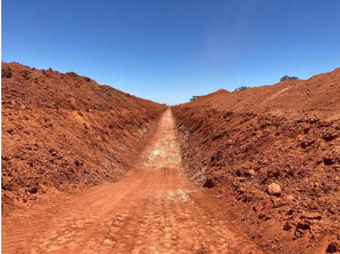
Plate 4: Overview of the West Cut-off trench – base.
