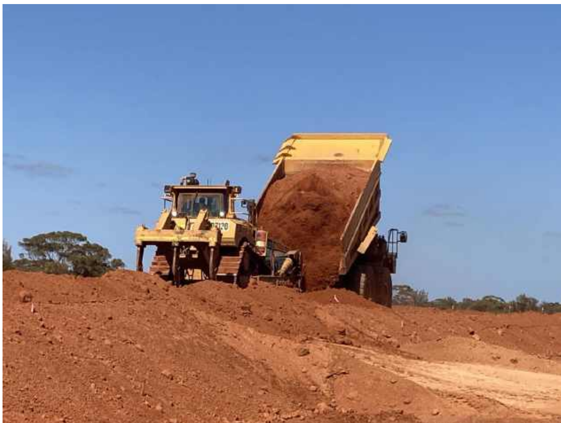
Plate 2: Dumping Zone C material, Cell 3 - South embankment, Layer – 3.
