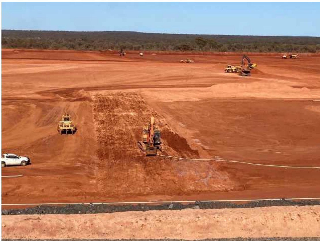
Plate 4: View of CSL Trial Pad while it was moisture conditioned.
