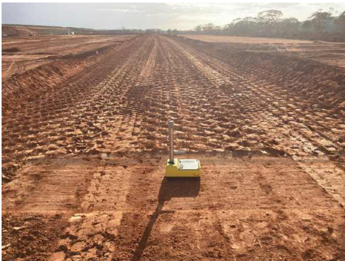
Plate 1: Field Density Testing, Cell 3 – South embankment, Layer – 4.
