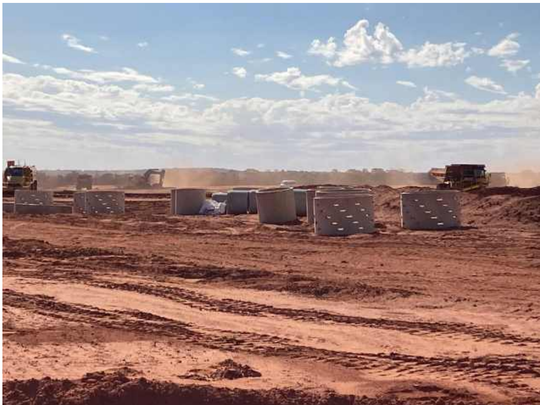
Plate 6: Overview of Laydown area for Decant & Underdrainage towers components.
