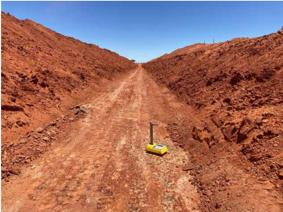
Plate 4: NDM compaction test at West Cut-off trench – base.
