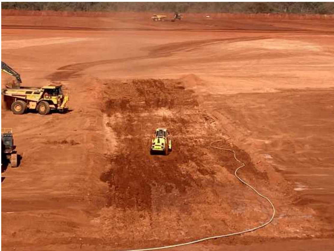
Plate 4: View of CSL Trial Pad while it was compacted.
