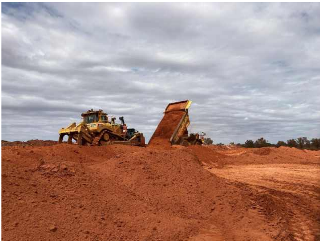
Plate 2: Dumping Zone C material, Cell 3 - North embankment, Layer – 3.
