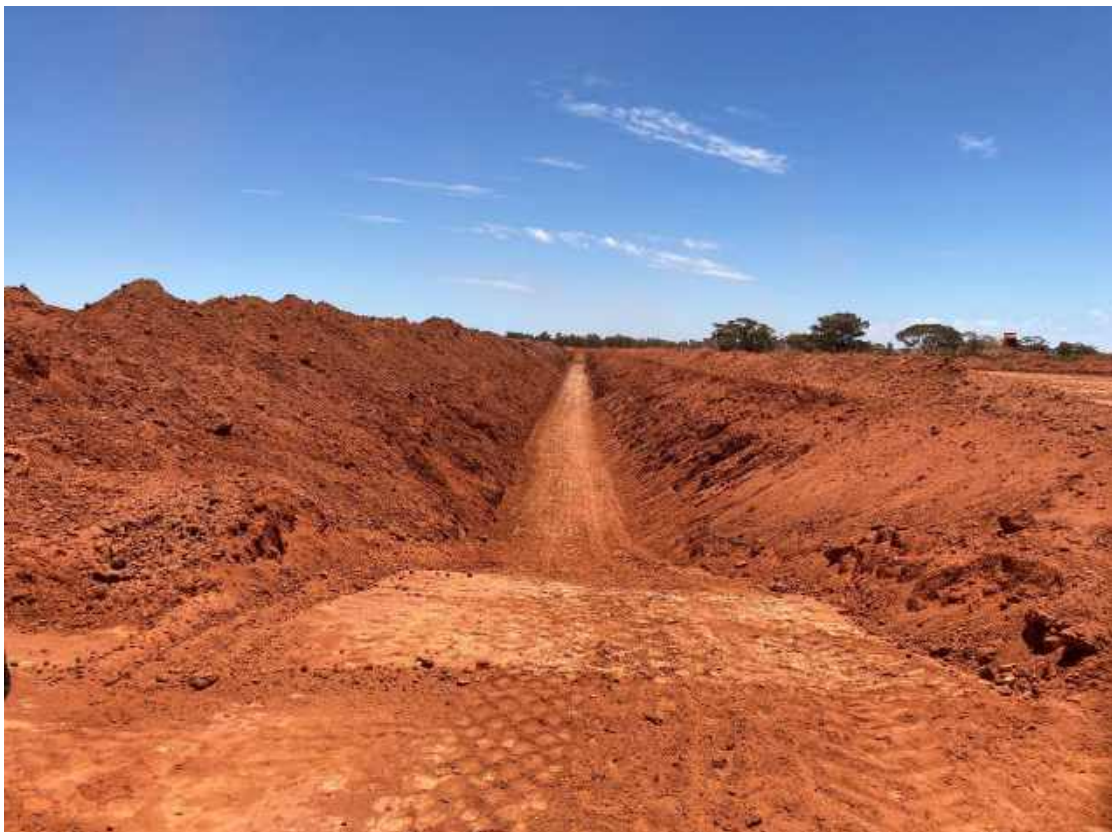
Plate 2: Overview of North Cut-off trench looking West.
