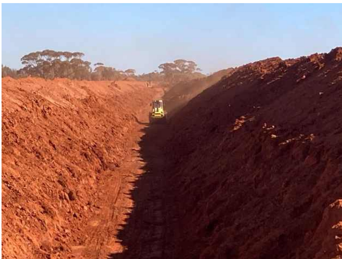
Plate 3: Compacting West Cut-off trench – base.
