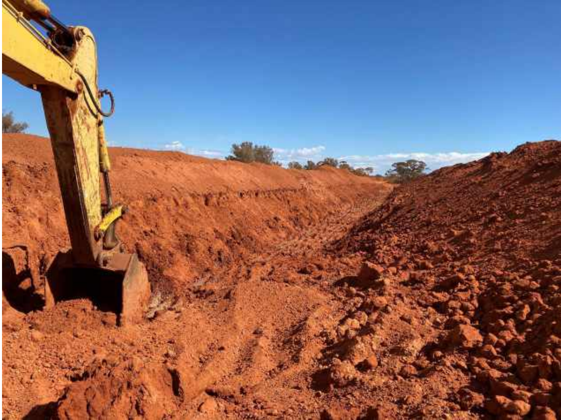
Plate 5: Excavating Cut-off trench ( \approx 4\text{m} deep or suitable depth) in West embankment.
