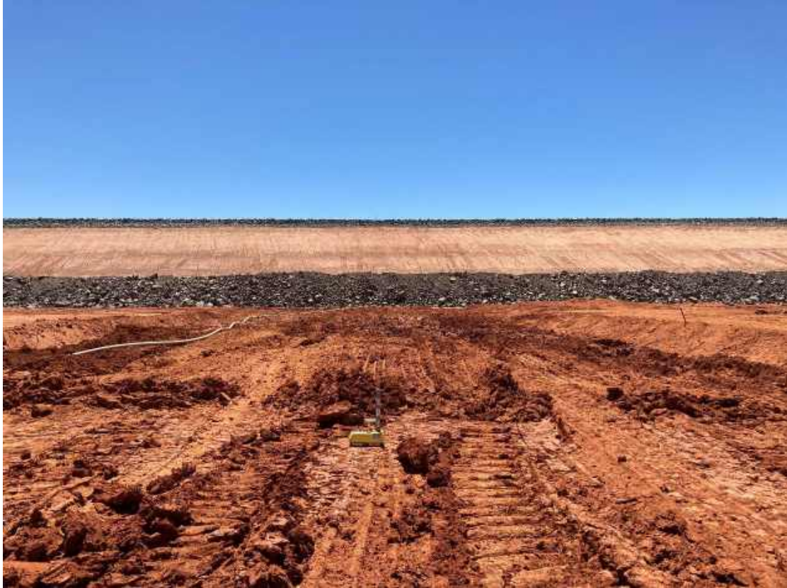
Plate 5: NDM Compaction test at CSL Trial Pad - Causeway location.
