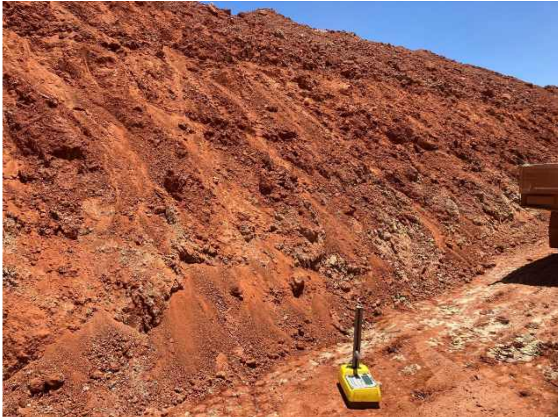
Plate 3: NDM Compaction test at North Cut-off trench - Zone A - base.
