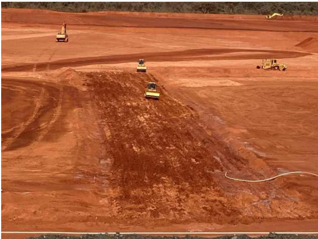
Plate 6: Rolling of CSL Trial Pad.
