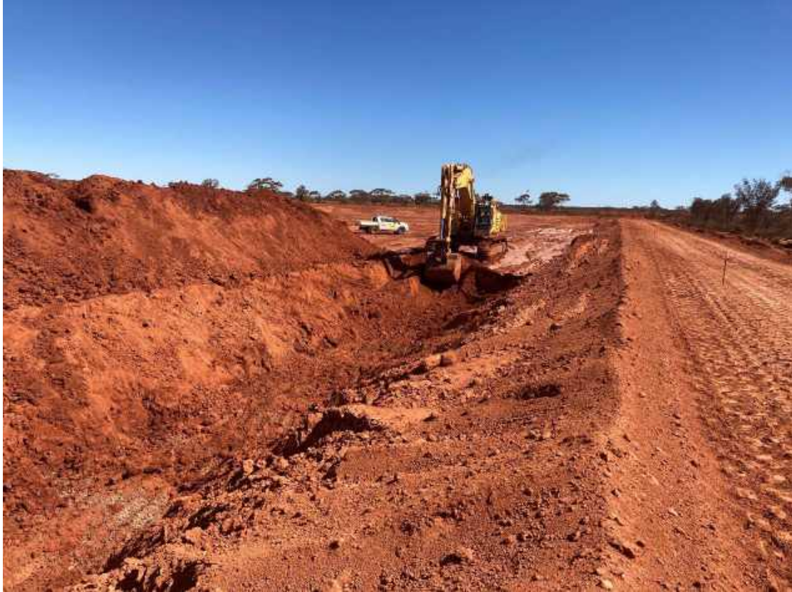
Plate 3: Excavating Cut-off trench ( \approx 4\text{m} deep or suitable depth) in West embankment.
