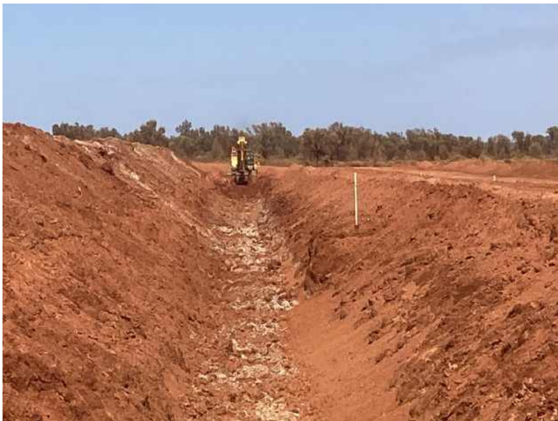
Plate 5: Excavating cut-off trench ( \approx 4\text{m} deep) in North embankment.
