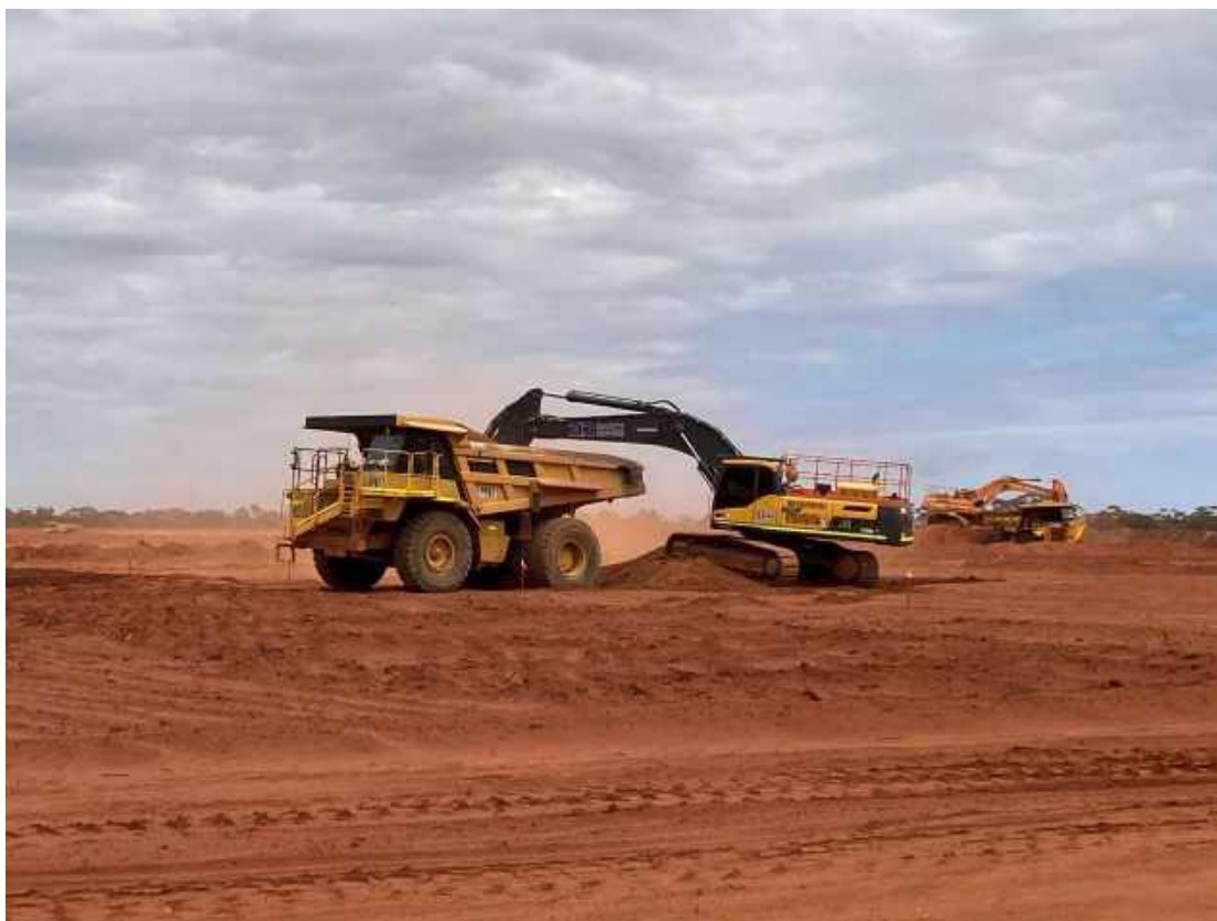
Plate 1: Loading Zone C material at borrow pit.
