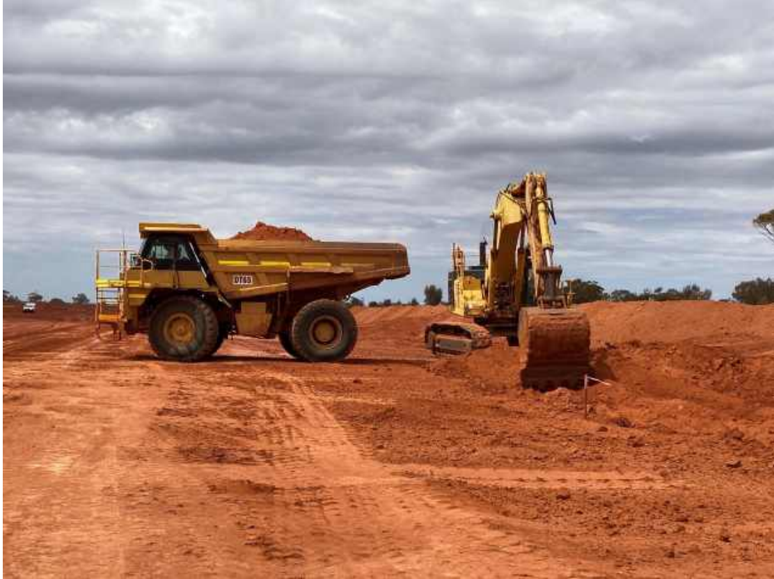
Plate 3: Excavating cut-off trench ( \approx 1\text{m} deep) in North embankment.
