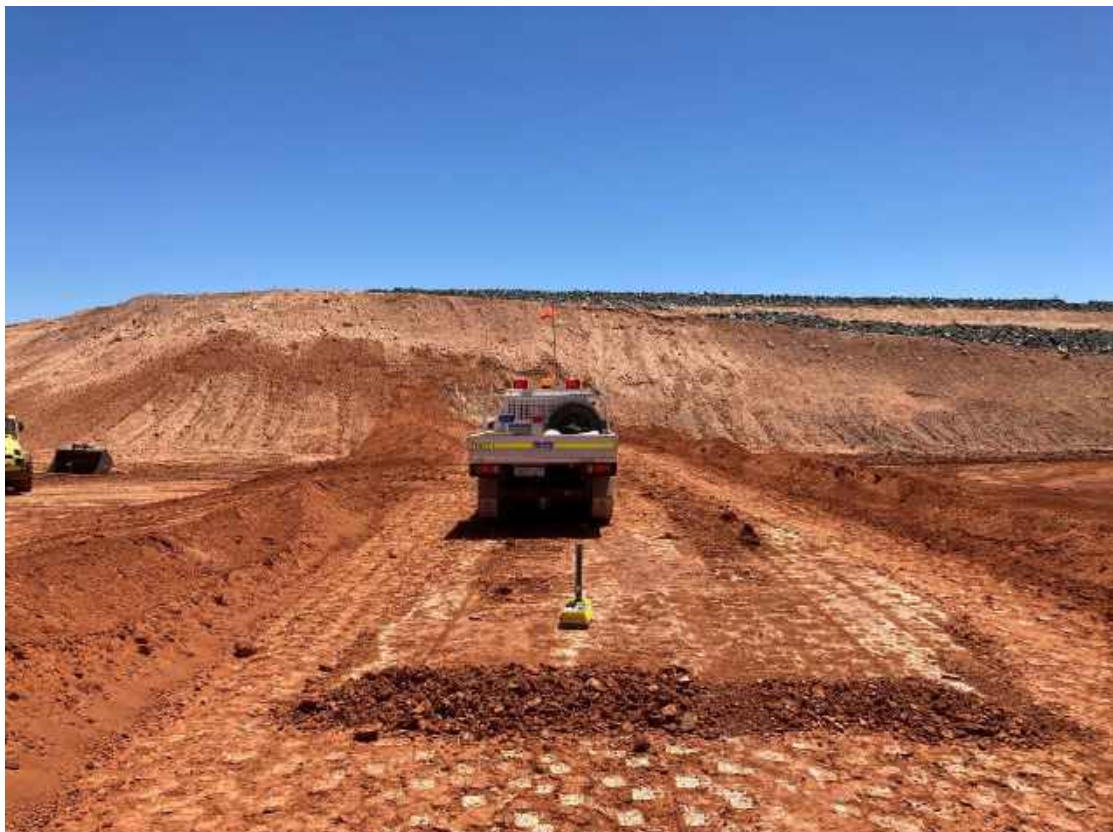
Plate 2: NDM Compaction test at South Embankment – Zone C – layer 4.
