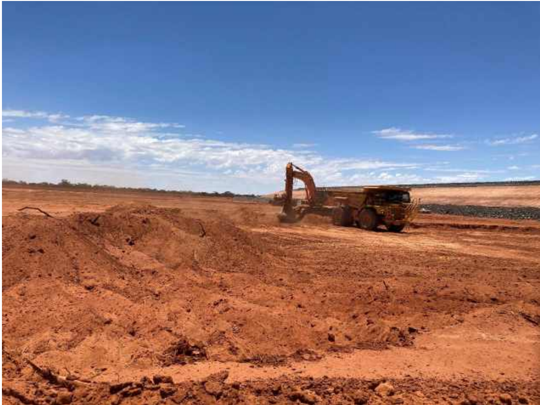
Plate 1: Loading Subsoil with vegetation at Causeway location.
