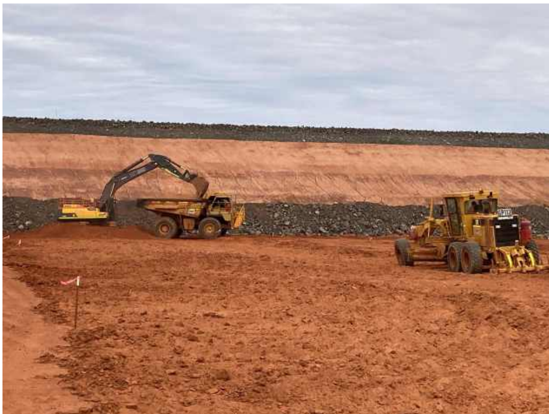
Plate 5: Causeway, excavating subsoil, removing just enough material to be clear of vegetation.
