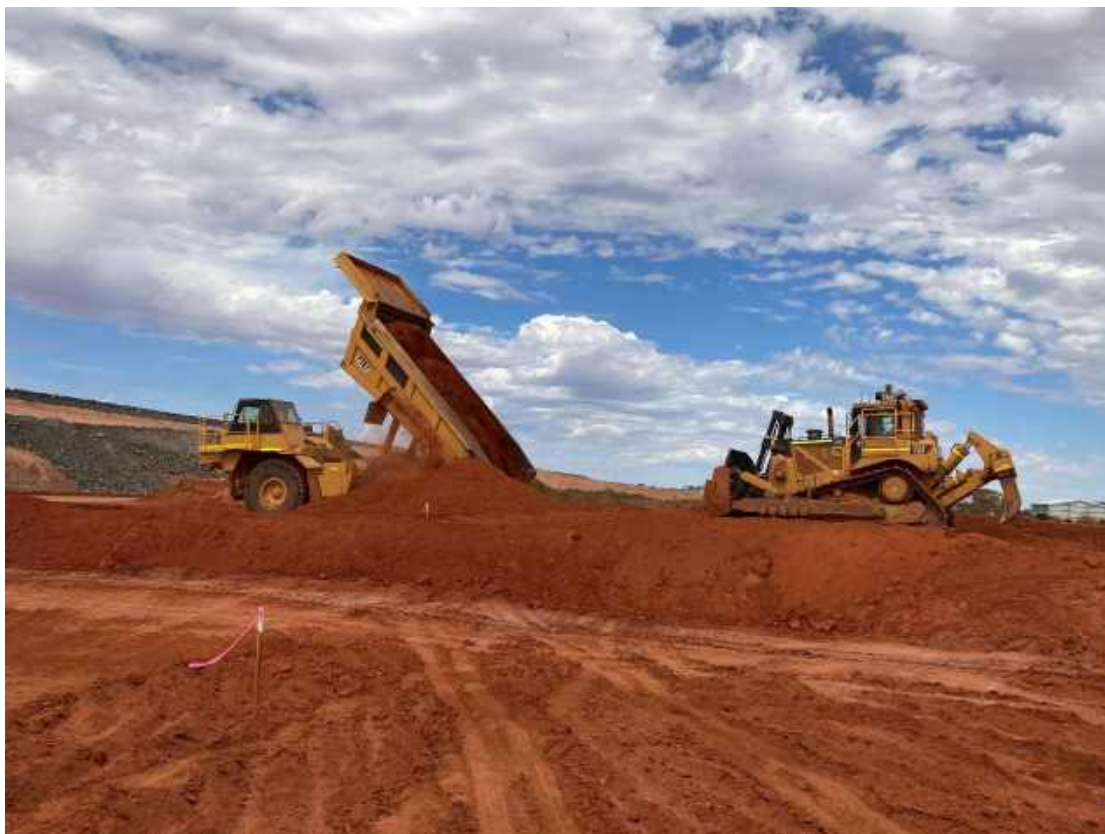
Plate 3: Dumping and spreading Zone C material at South Embankment - layer 2.
