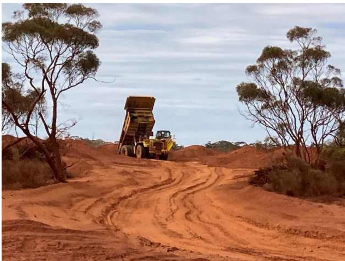
Plate 6: Dumping subsoil material with vegetation at designated stockpile area.
