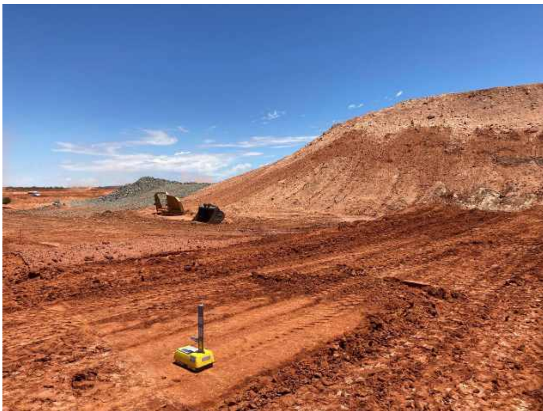
Plate 4: NDM Compaction test at South Embankment – Zone C – layer 2.
