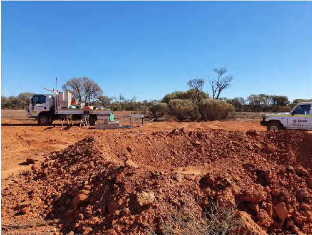
Plate 1: C-BH05 – Location – North
