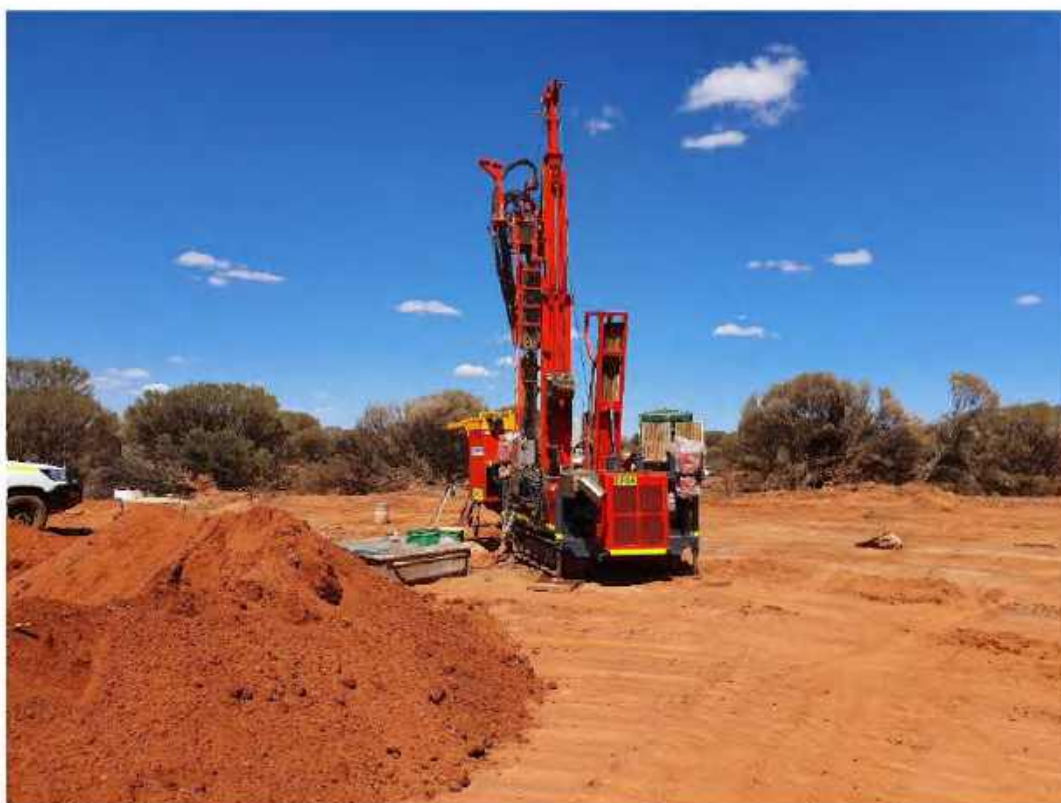
Plate 68: C-BH07 – Location – South
