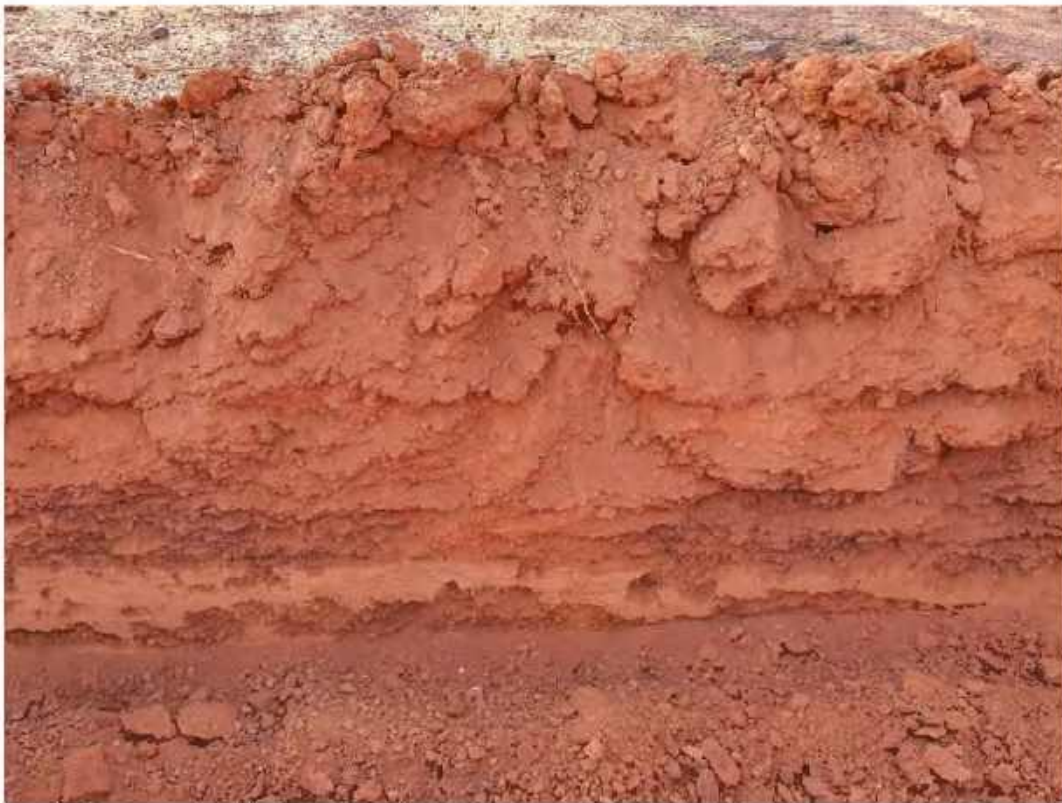
Plate 18: C-TP-39 – Test Pit
