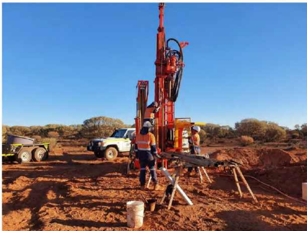
Plate 32: C-BH06 – Location – North
