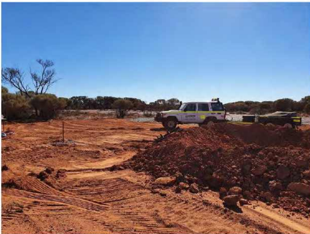
Plate 2: C-BH05 – Location – East
