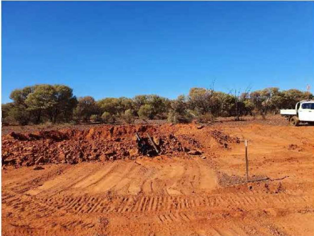
Plate 3: C-BH05 – Location – South
