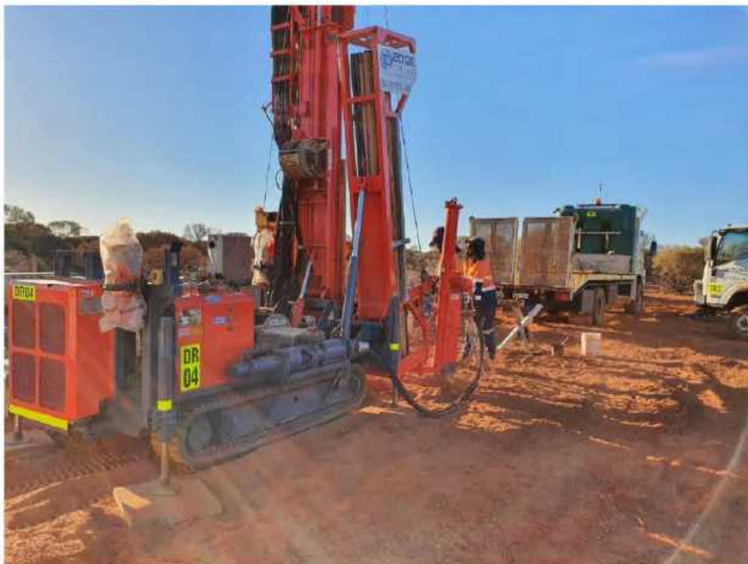
Plate 34: C-BH06 – Location – South
