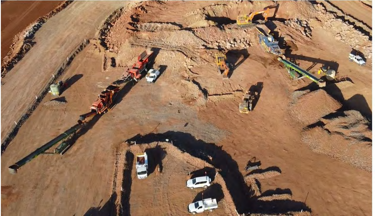
Figure 4 - As of 20 January 2024, crushing and screening circuits at Site C
