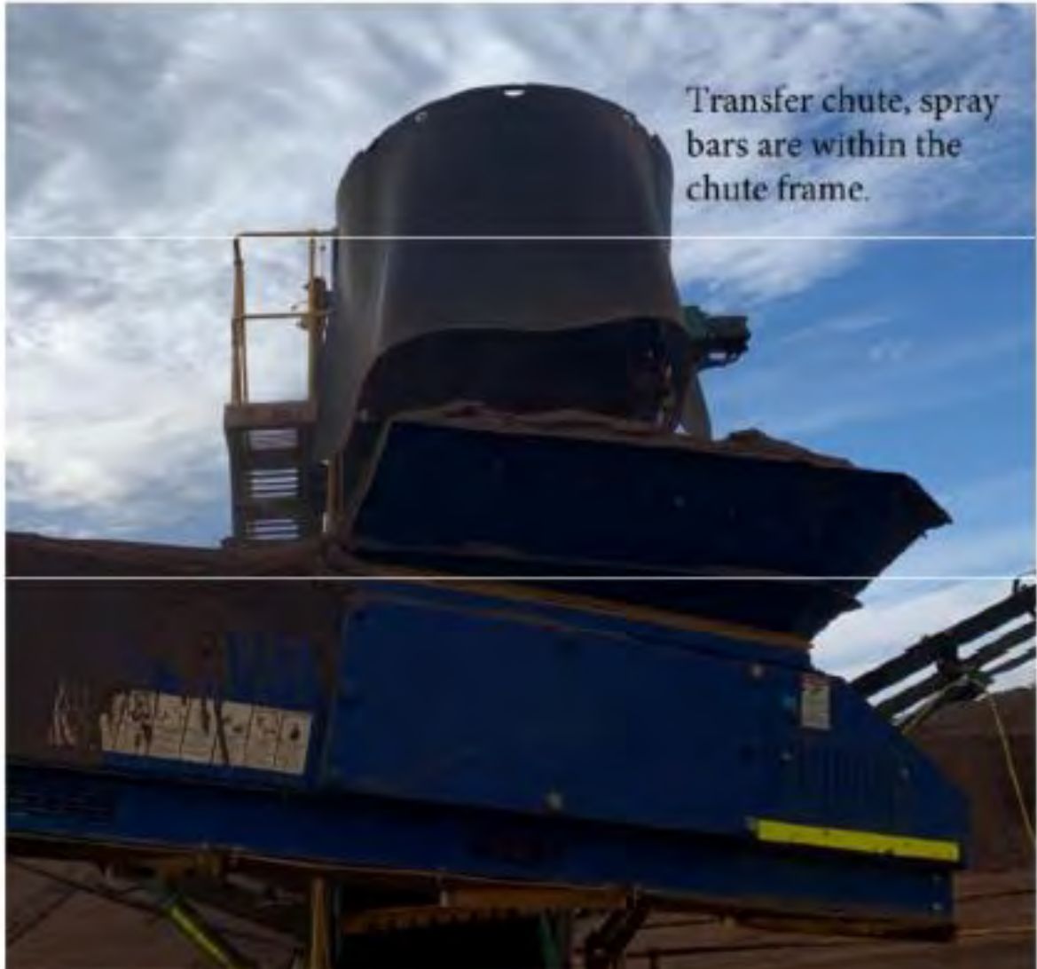
Figure 33 - Transfer Chute with dust controls
