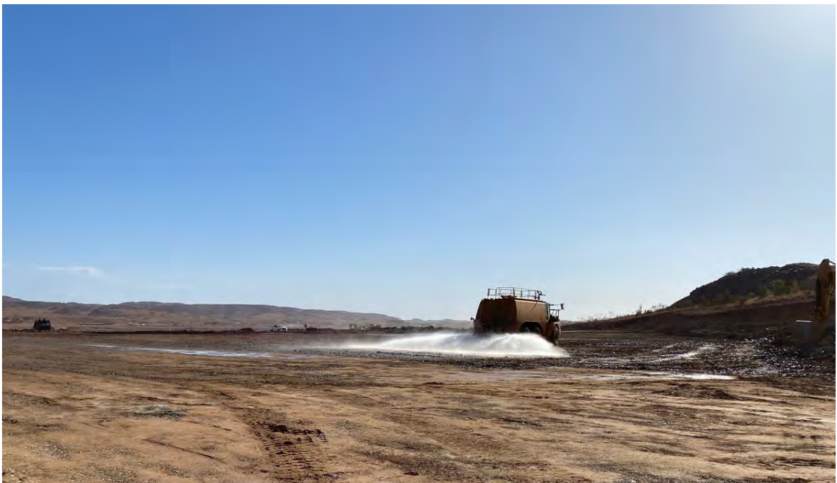
Figure 14 – Water Cart in use on Site C, 20 January 2024
