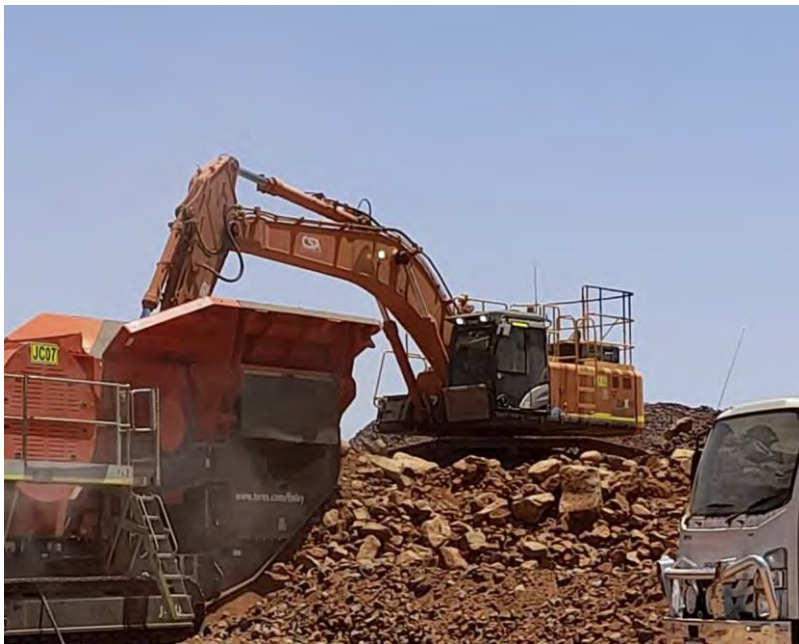
Figure 11 – Supporting equipment - Hitachi ZX490lc-5 excavator.
