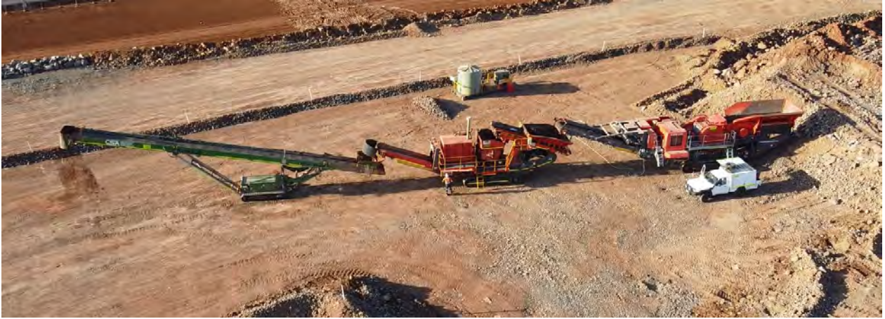
Figure 6 - As of 20 January 2024, crushing and screening circuits at Site C
