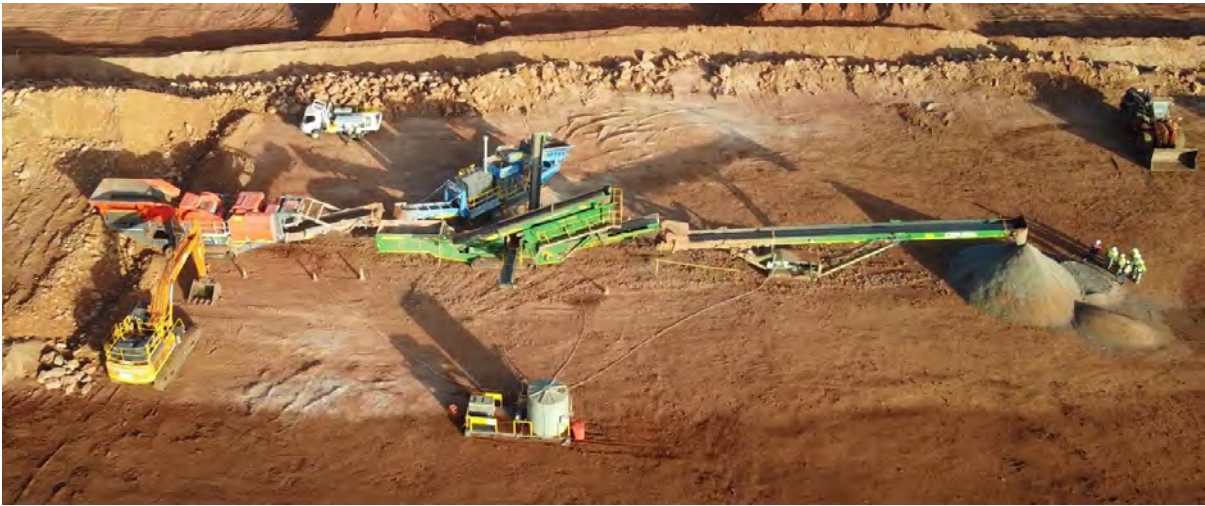
Figure 7 – As of 19 January 2024, crushing and screening circuits at Site F
