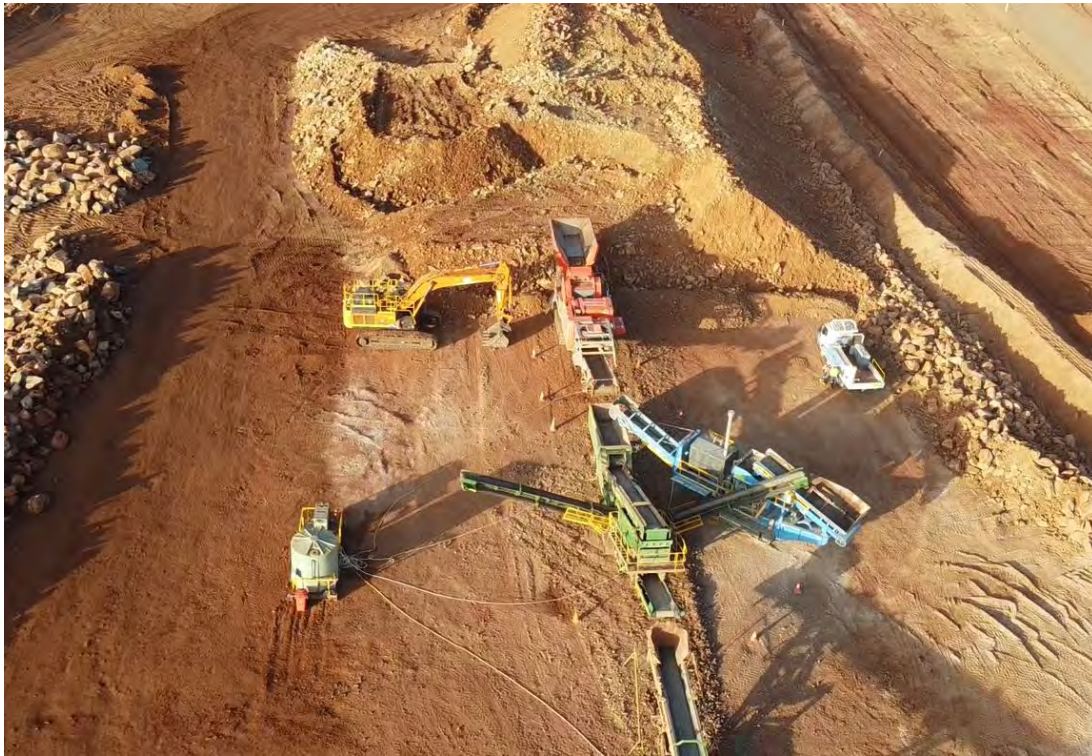
Figure 9 – As of 19 January 2024, crushing and screening circuits at Site F
