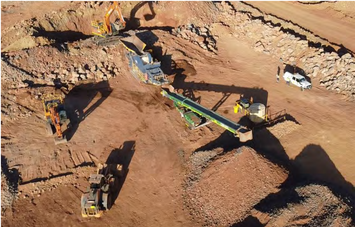
Figure 5 - As of 20 January 2024, crushing and screening circuits at Site C
