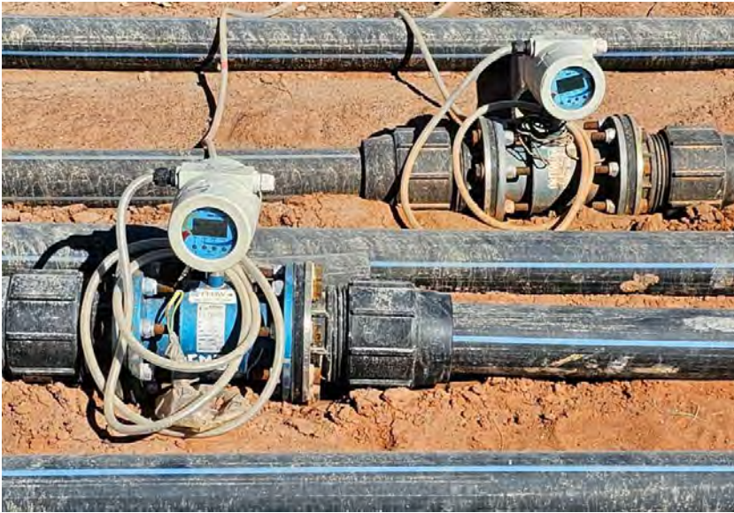
Figure 2: Photo of dewatering flowmeters at tag board
