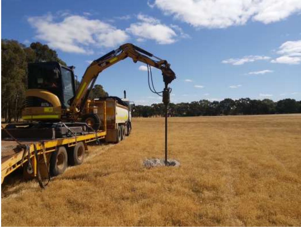
Photo 05: Subsurface probing at Bore Hole (BH5) by mechanical auger
