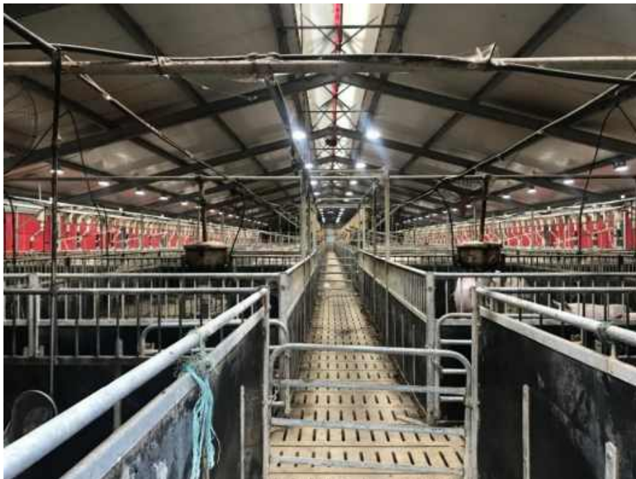
Figure 9. Inside a shed with concrete slatted flooring.
