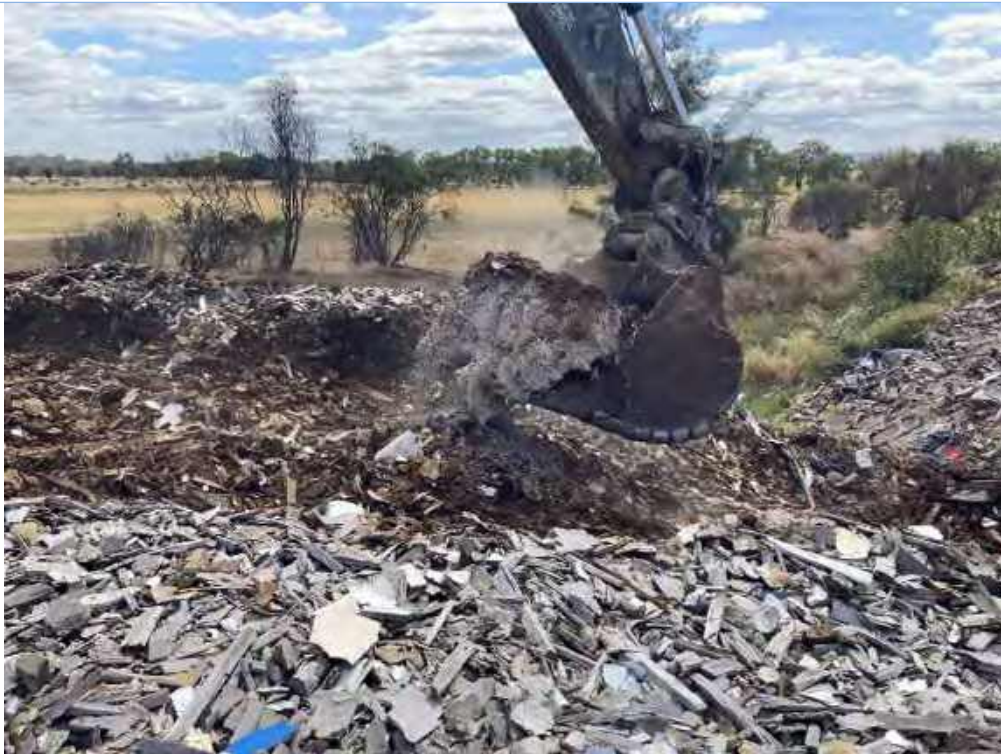
Photograph 8: Wood material found within test pit location WC07 (refer to Figure 4).
