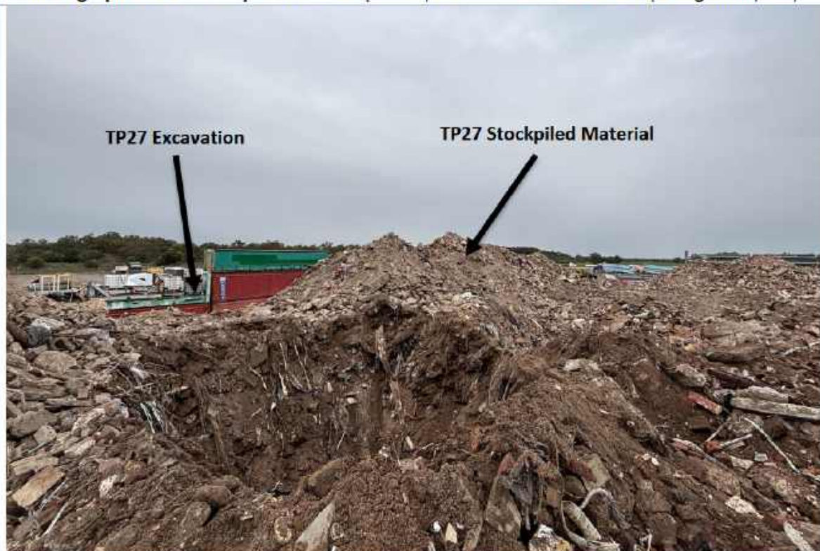
Photograph 4: TP27 stockpiled material (centre) and TP27 excavated area (background, left).
