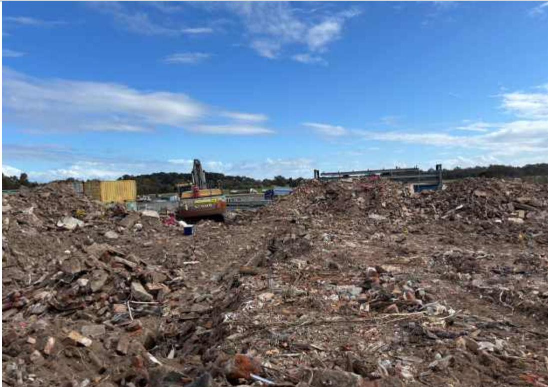
Photograph 2: Surface conditions of the Main Stockpile, note 20t excavator in background.
