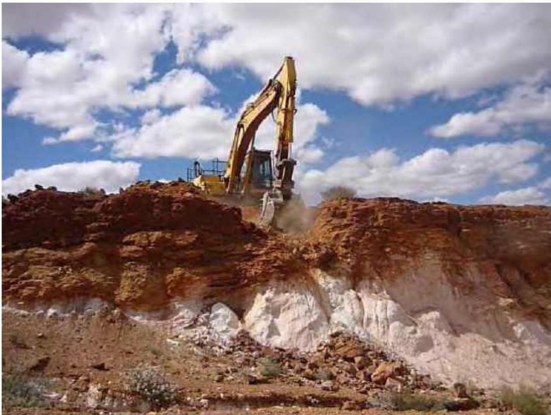
Photograph 6: Ripping trial of laterite zone (3/02/2012)
