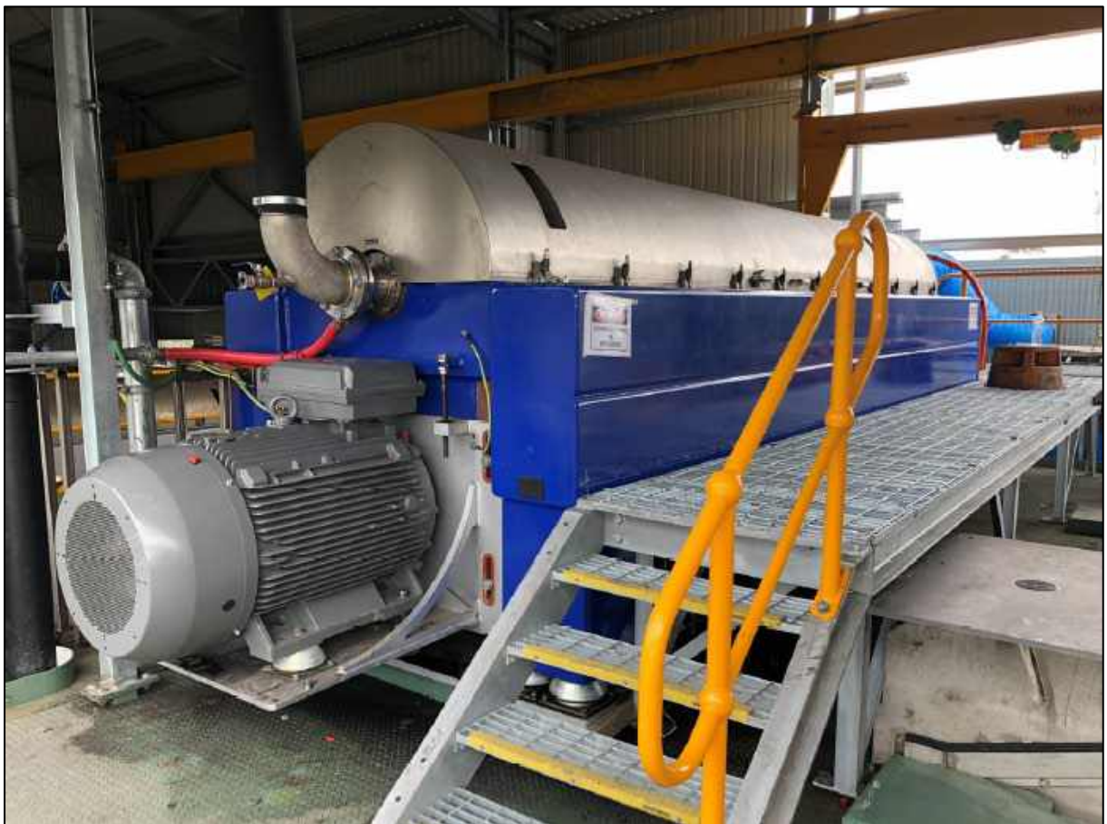
Plate 5-4: Decanter Centrifuge Unit
