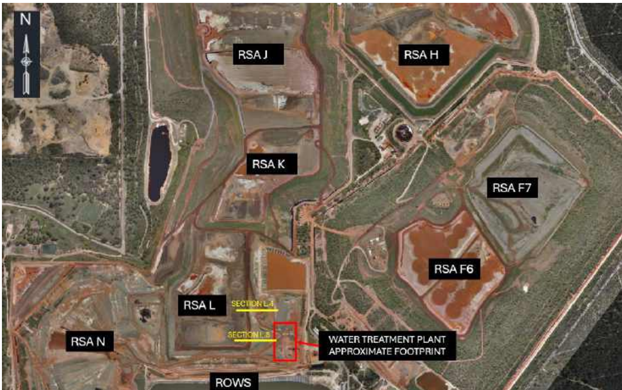
Figure 1-1 Approximate footprint of WTP hardstand indicated by red rectangle
