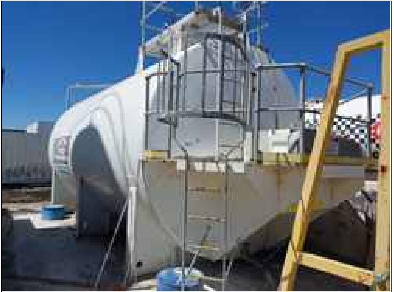
Plate 1: Milk of Lime Dosing System
