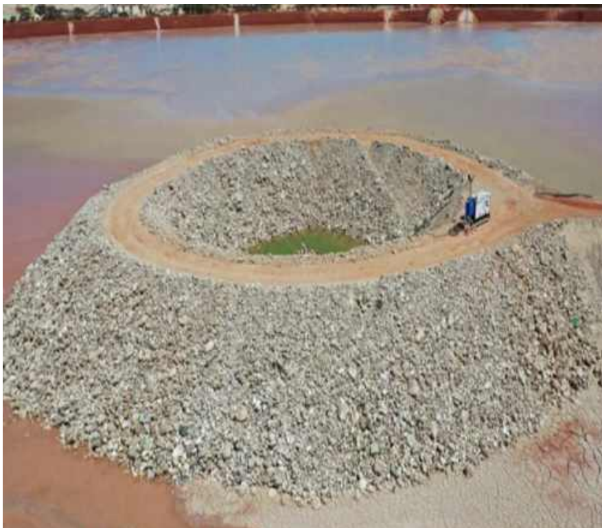
Figure 24: Example of a rock-ring decant structure
