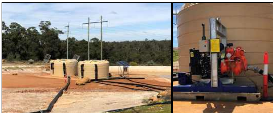
Figure 7 and Figure 8: Drainage site 2 Sykes CPT100i pump
