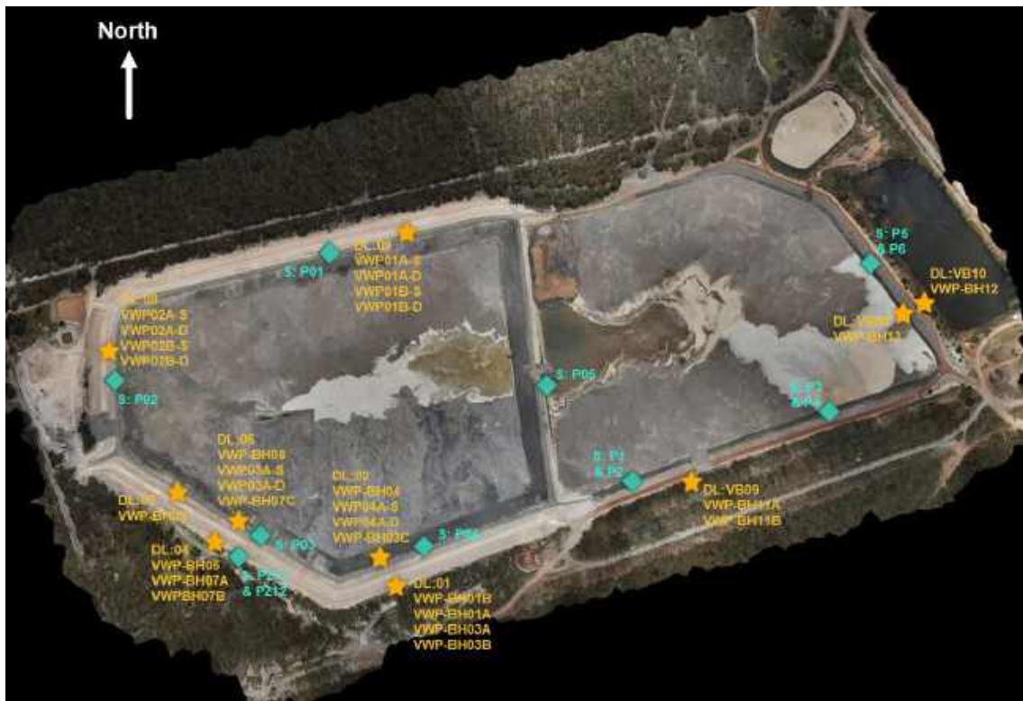
Figure 34: FAD vibrating wire and manual dipping piezometers cells 1 and 2
