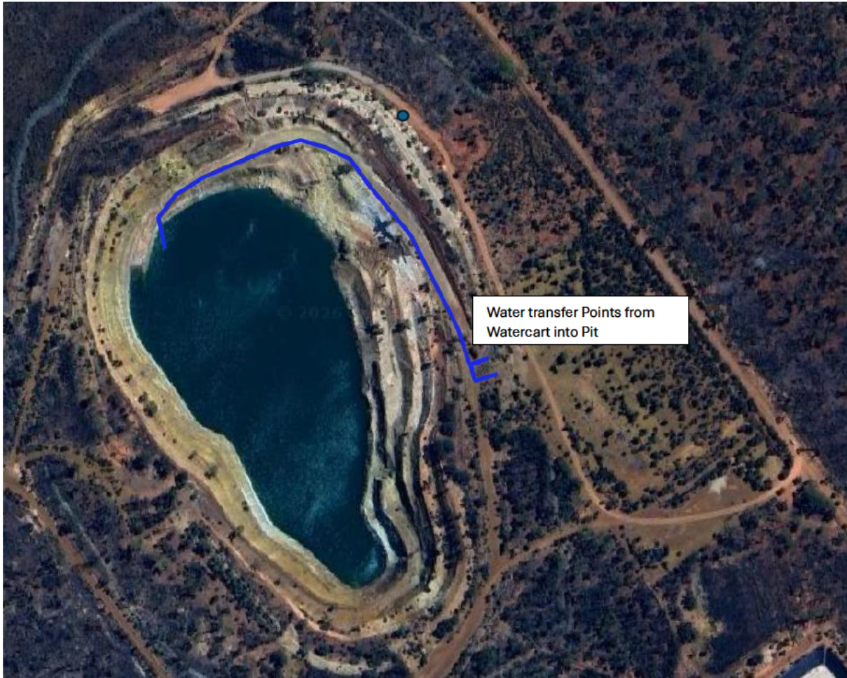
Shown above is the Diggers pit and pipeline location for watercarts to transfer into.
