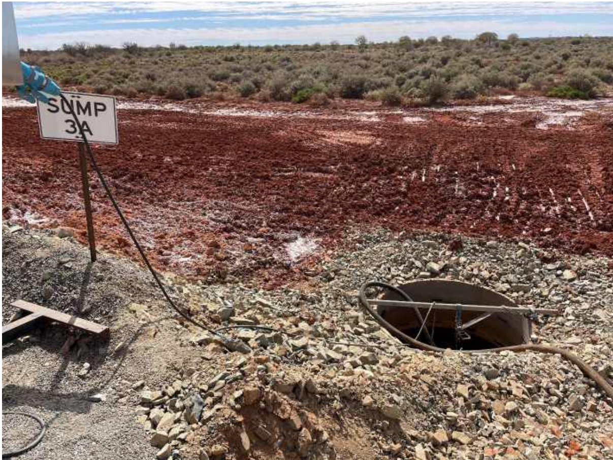
Figure 3: TSF sump installation (TSF SP03)
