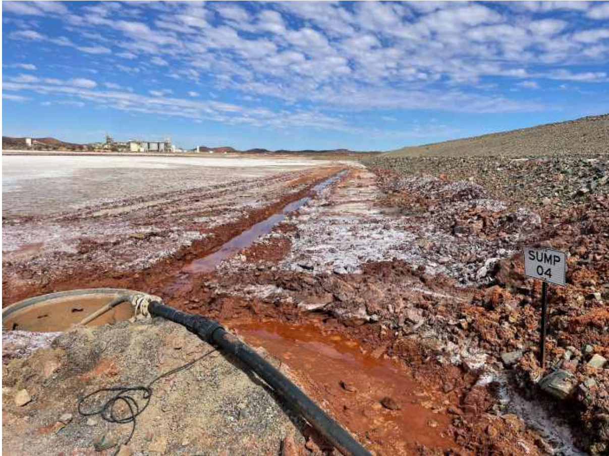
Figure 4: TSF sump with shallow drainage channel.
