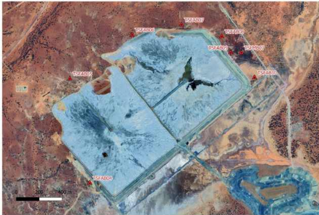
Figure 1-2 Locality of the TSF bores (marked in red) at the Mount Morgans TSF Project
