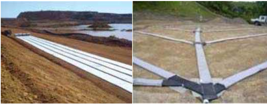
Figure 8-4 Megaflo panel drain examples (courtesy Geofabrics Australia)
