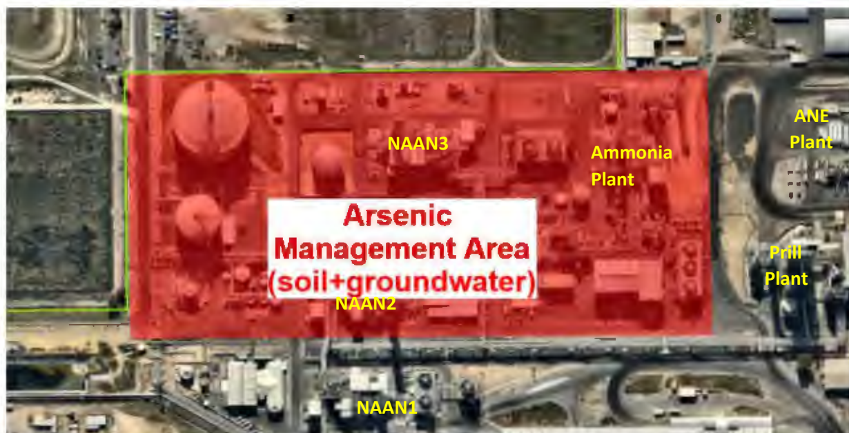
Figure 18: Arsenic Management Area (from Contaminated Site Management Plan)
