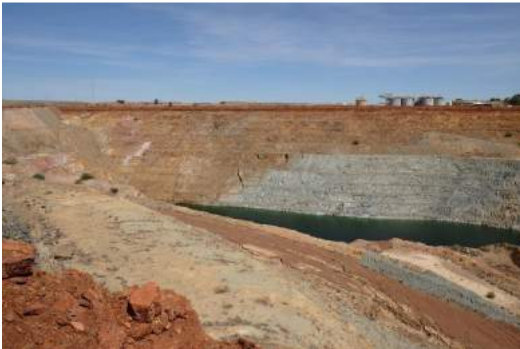
Figure 5 - GNH Pit west wall from east side (left of frame is adjacent to GNH)
