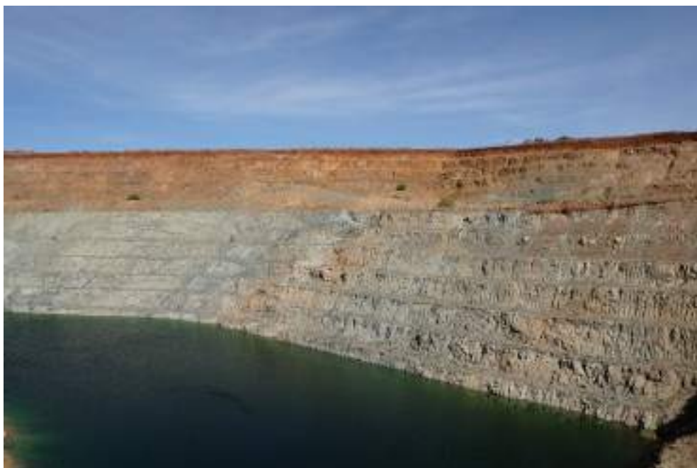
Figure 3 - West Wall of GNH Pit from north end
