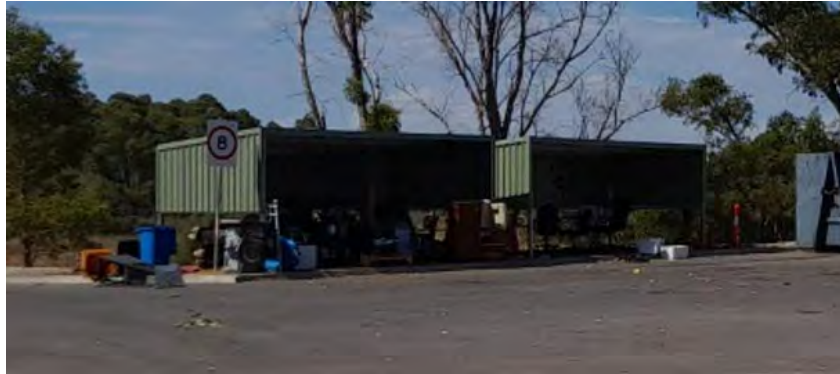
Existing shade structures.
