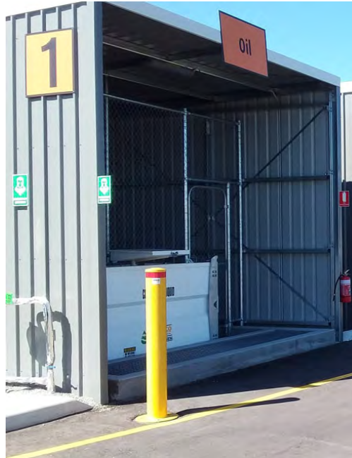
Malaga Recycling Centre – Oil Collection Shed.
