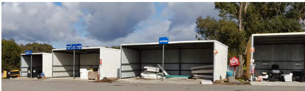
Existing collection shed example – Bullsbrook.
