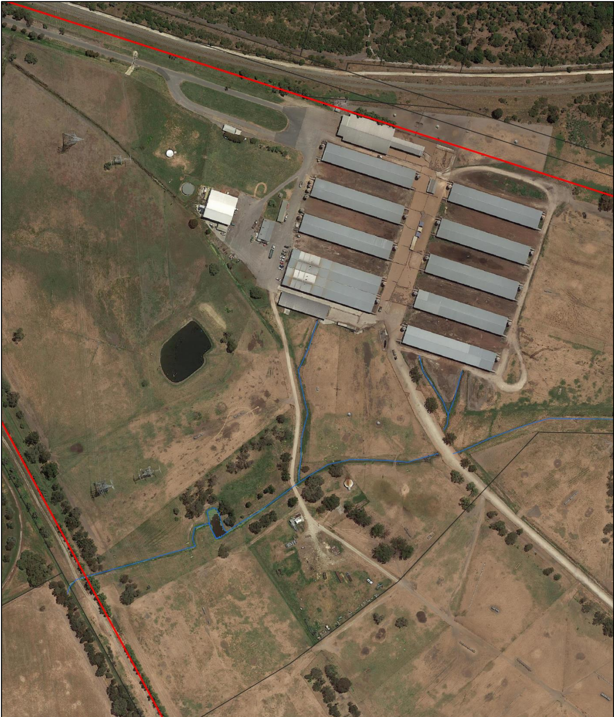
▲ Figure 1: Historical drain (blue line) was noted as being used to divert surface water runoff from the holding pens for off-site discharge, which is not authorised by the existing licence.
