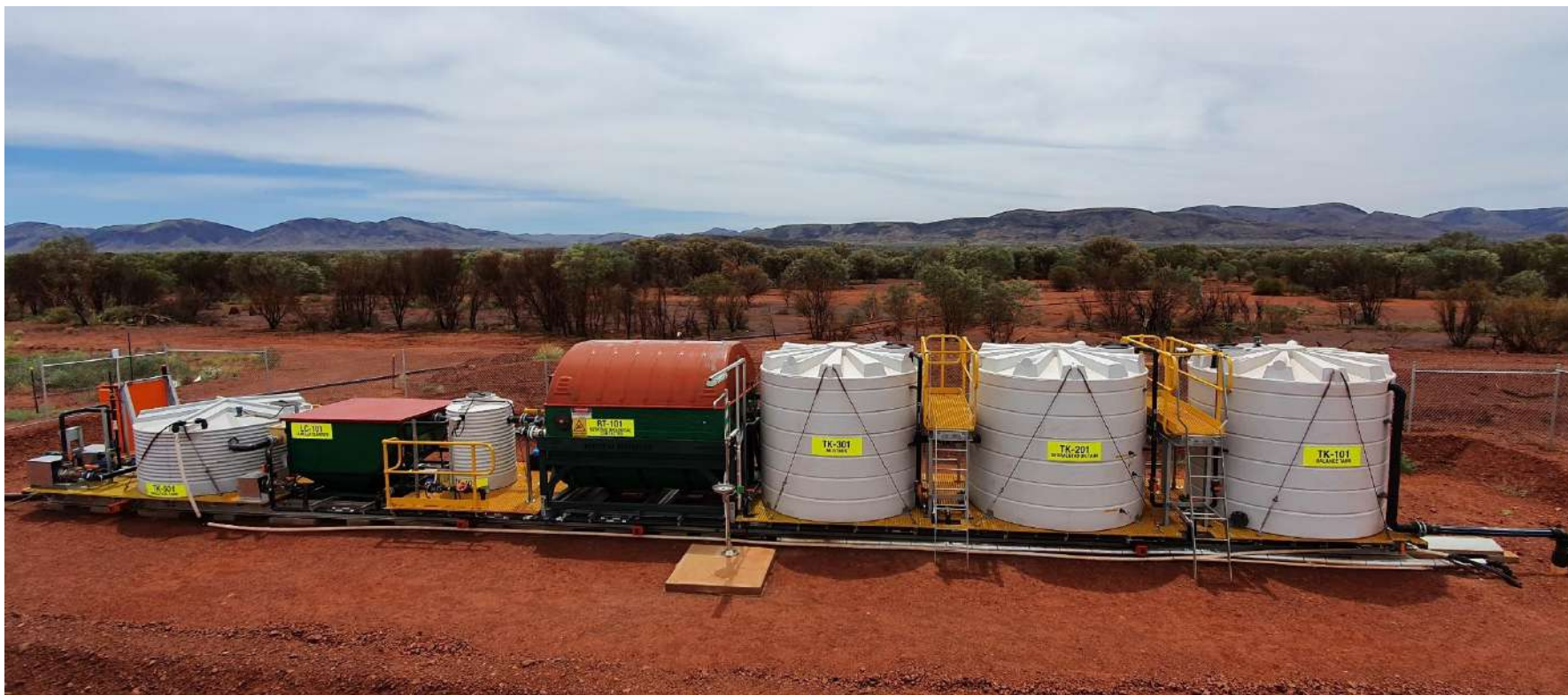
Figure 3: Evidence of Compliance – balance tank, sedimentation tank, Mixed Liquor recycle tank, RBC tank, Break tank, clarifier and treated effluent tank
