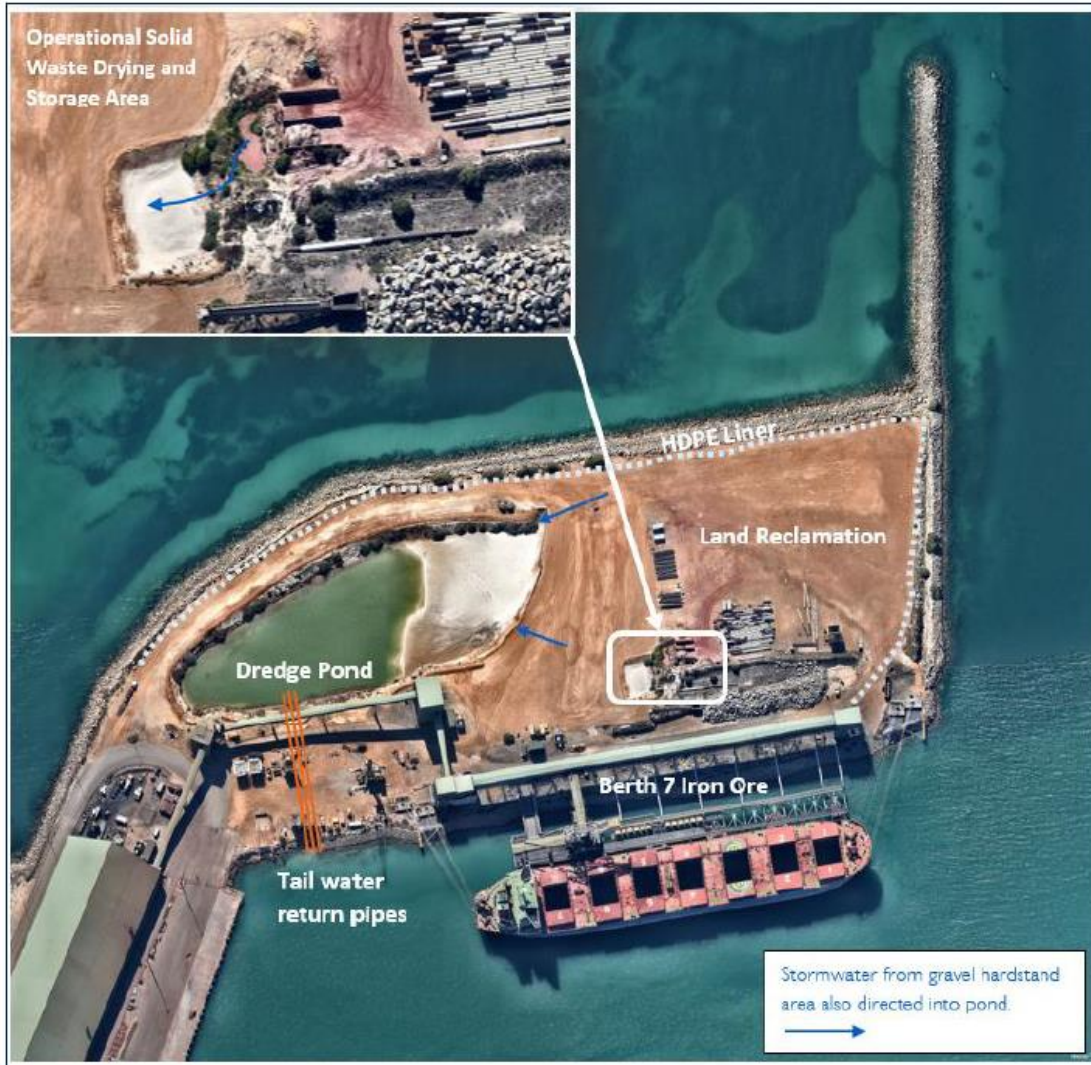
Figure 6: Location of dredge pond, tail water return pipe, and solid waste drying and storage area at Berth 7
