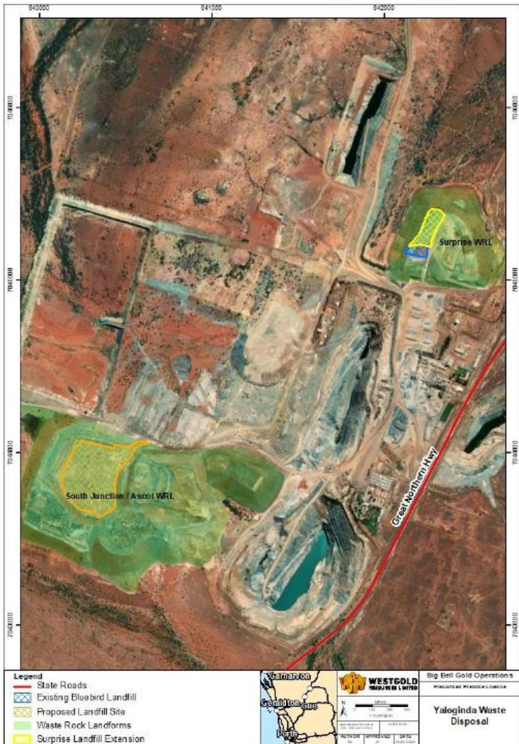
Figure 2: South Junction/Ascot WRL landfill and Surprise WRL landfill
