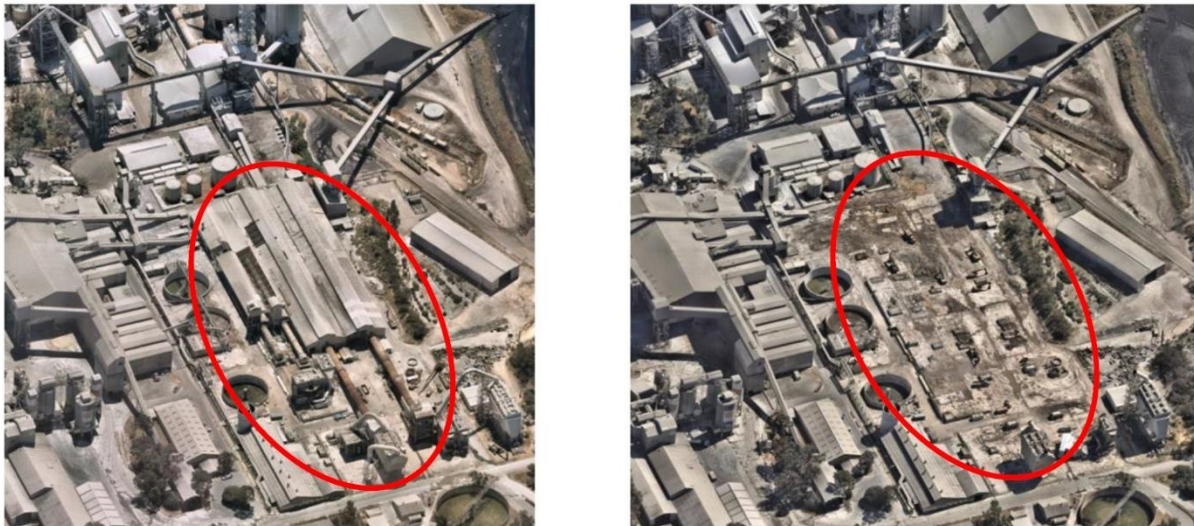
Figure 1: Kiln 3 and 4 before and after demolition
