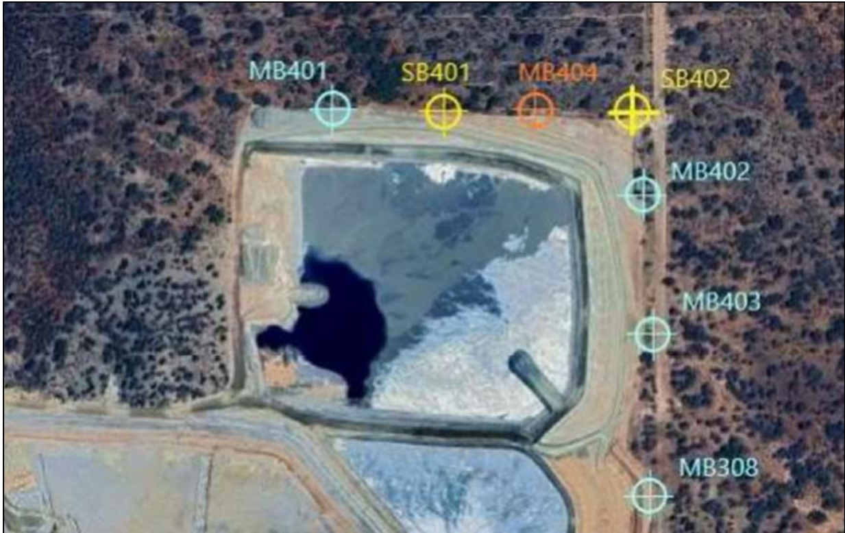
Figure 2: Location of existing groundwater monitoring bores (blue), new monitoring bores (orange), and new seepage recovery bores (yellow) at TSF4
