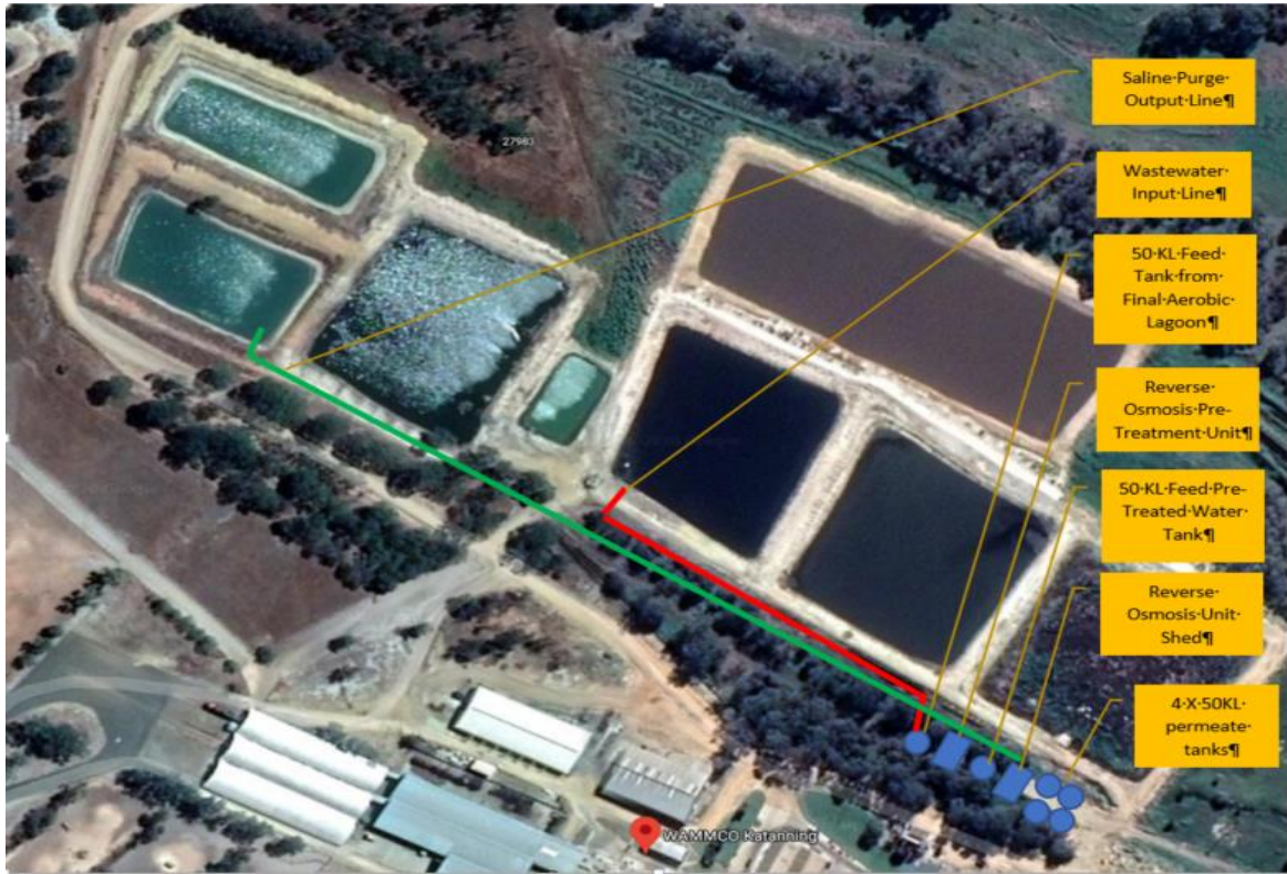
Figure 4: Reverse osmosis plant and associated infrastructure
