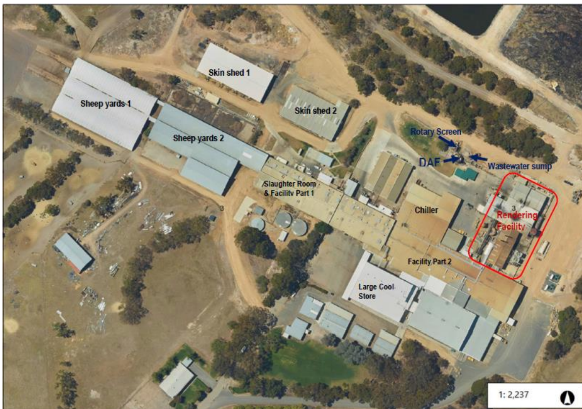
Figure 2: WAMMCO Katanning Abattoir key infrastructure
