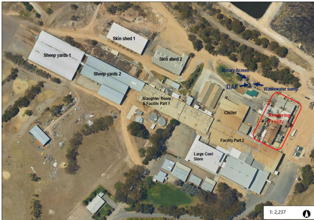
Figure 2: WAMMCO Katanning Abattoir key infrastructure
